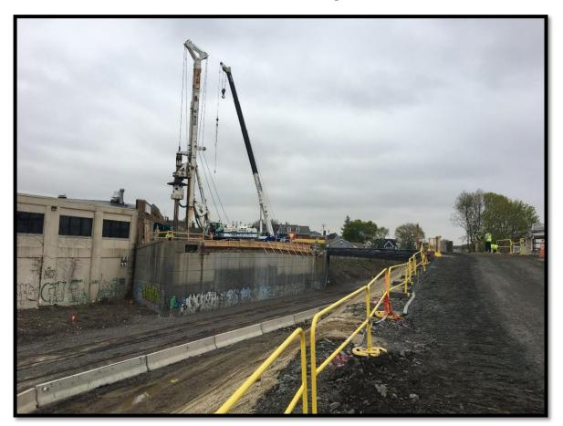
Temporary shoring for foundation work on the new bridge continues on the east side of the alignment
