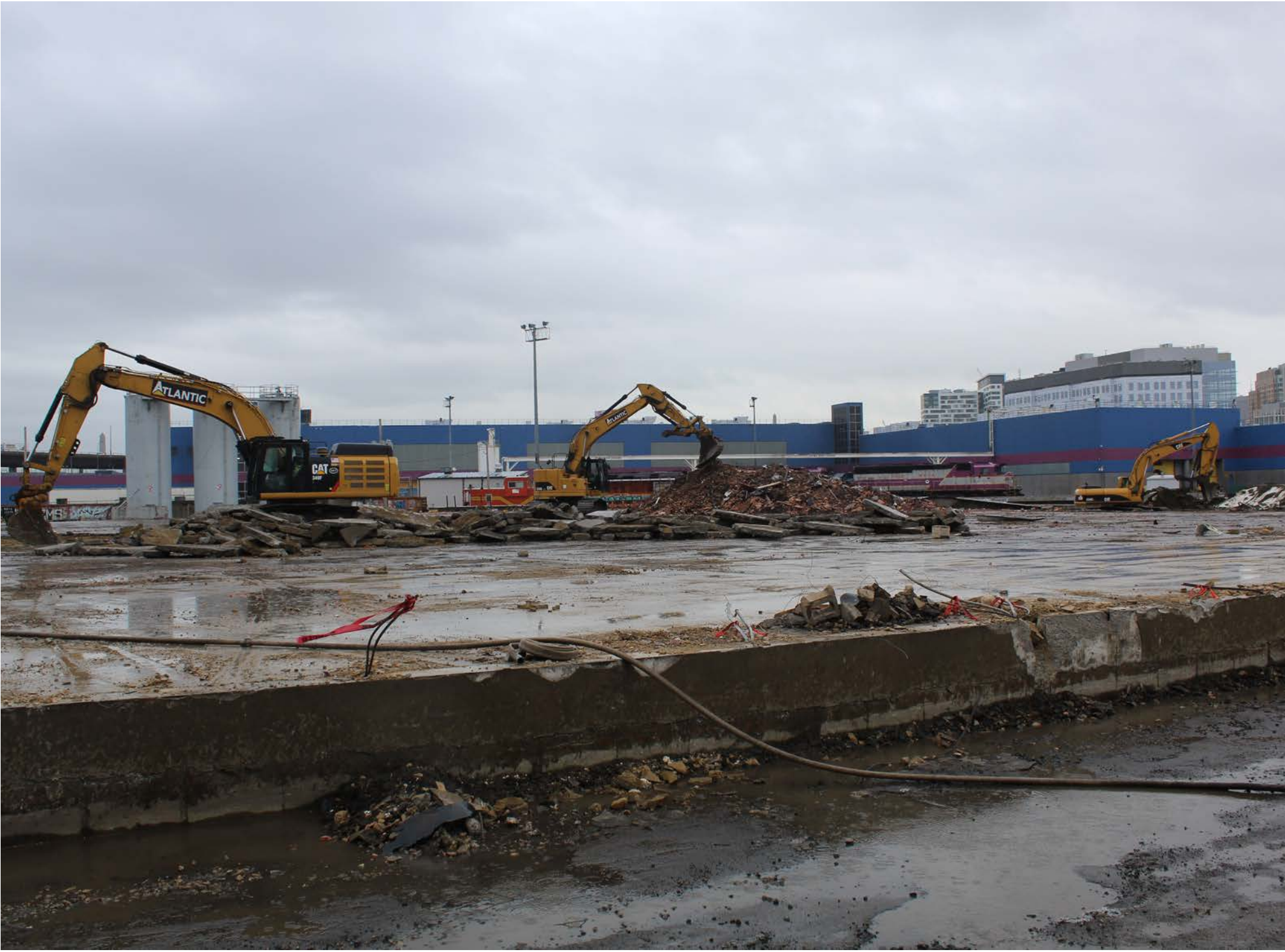
Backhoes' size reduce demolition debris (February 2019)
