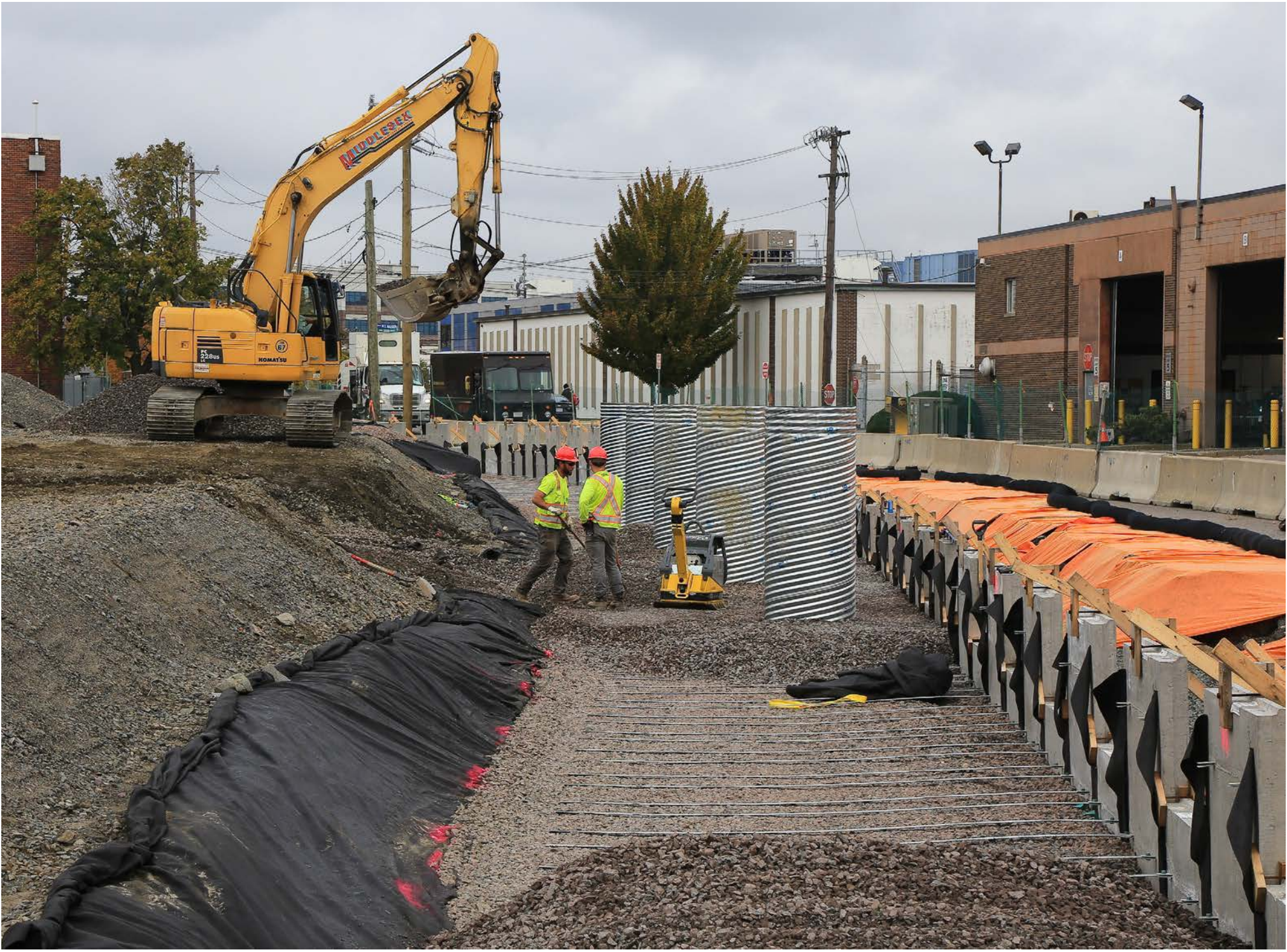
Retaining wall and drainage being built around the 3.25 acre complex (October 2019)
