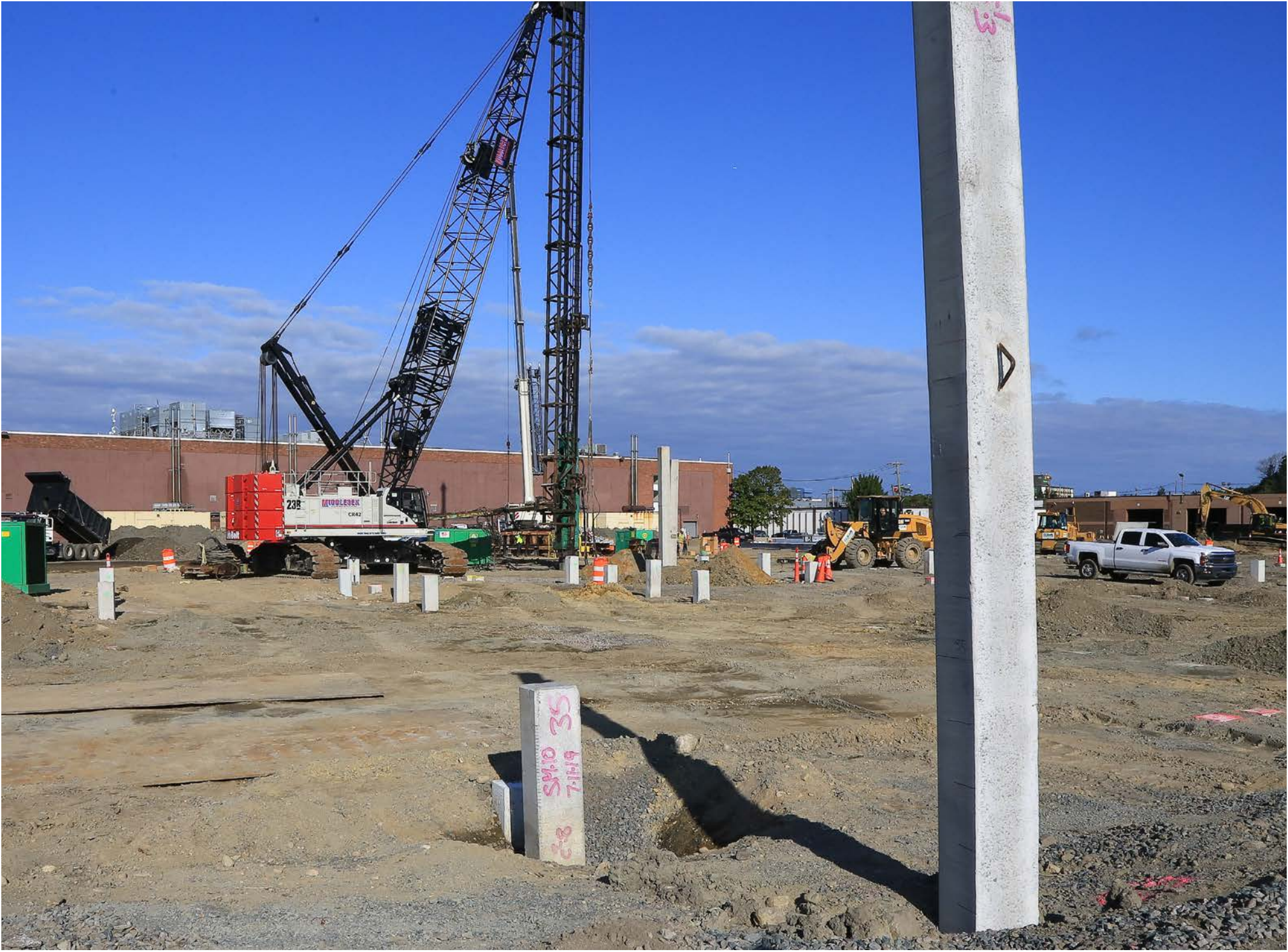
276 concrete piles were driven in for VMF foundation (Sept. 2019)
