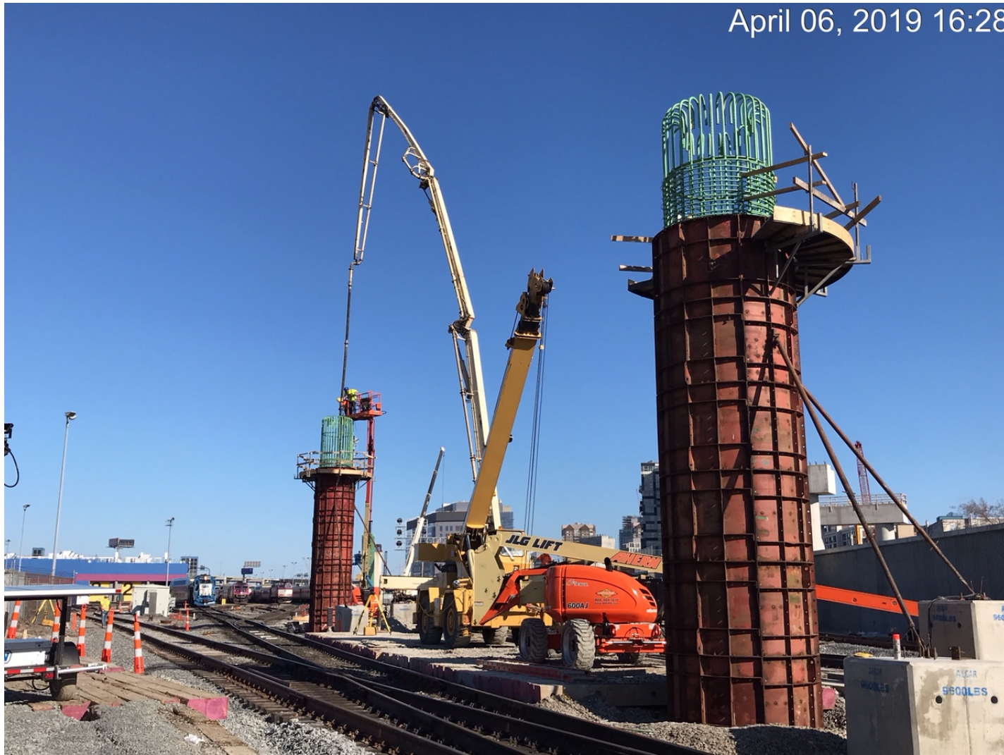
Viaduct Column Installation
