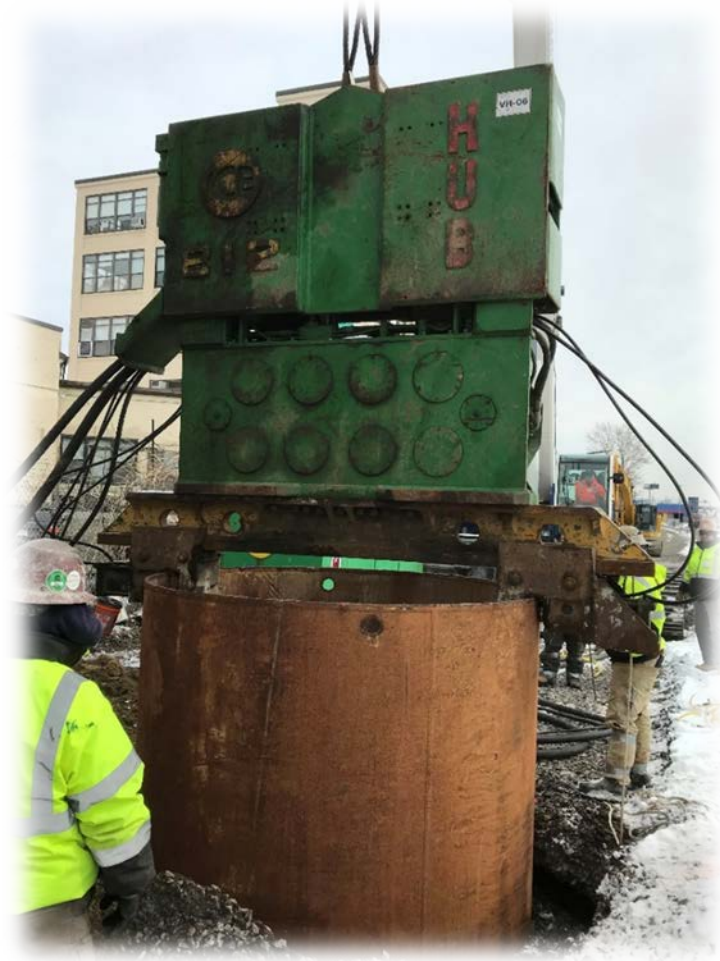
Viaduct Drilled Shafts
