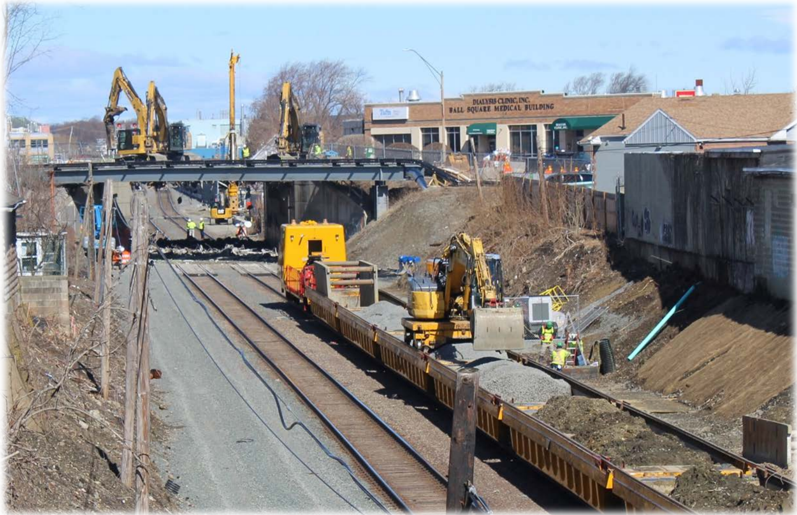
Multi-Purpose Machine (MPM®), drainage installation, bridge demolition, noise wall work
