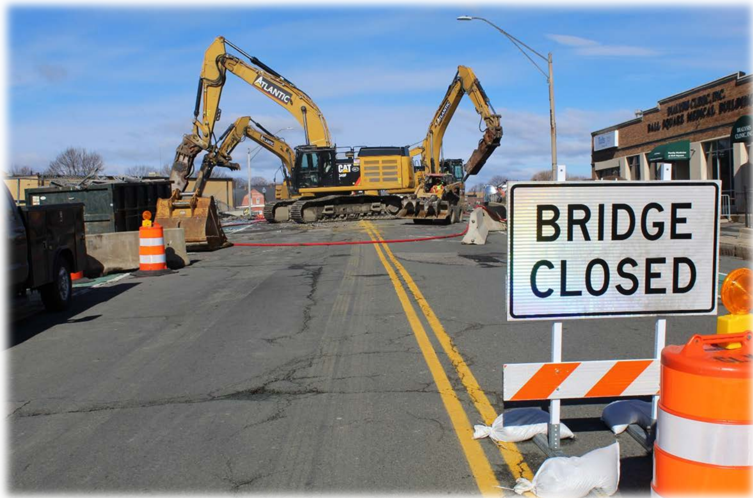
Broadway Bridge deck demolition
