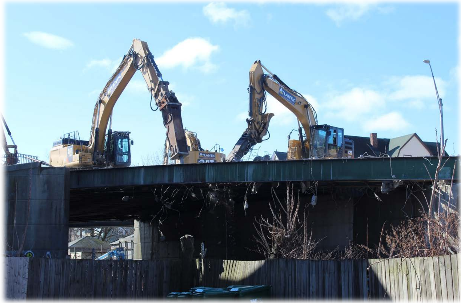
Broadway Bridge deck demolition
