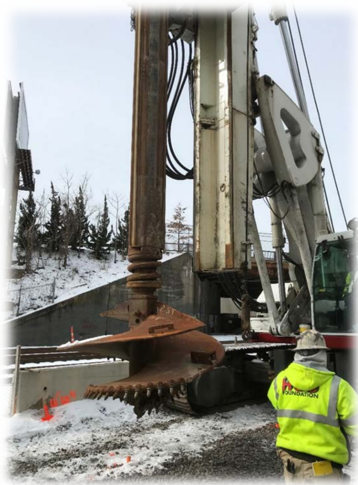
Viaduct Drilled Shafts
