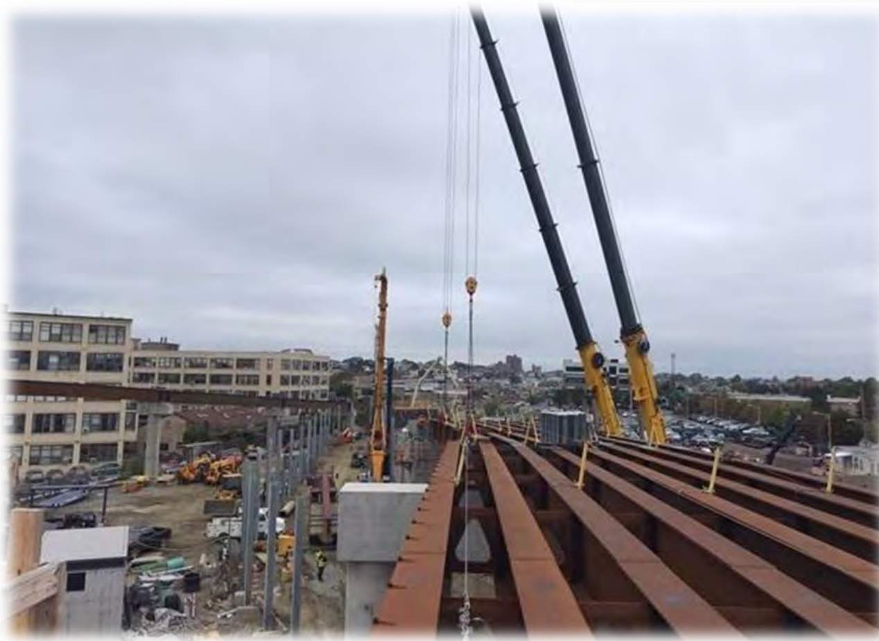
Final Span of viaduct structural steel
