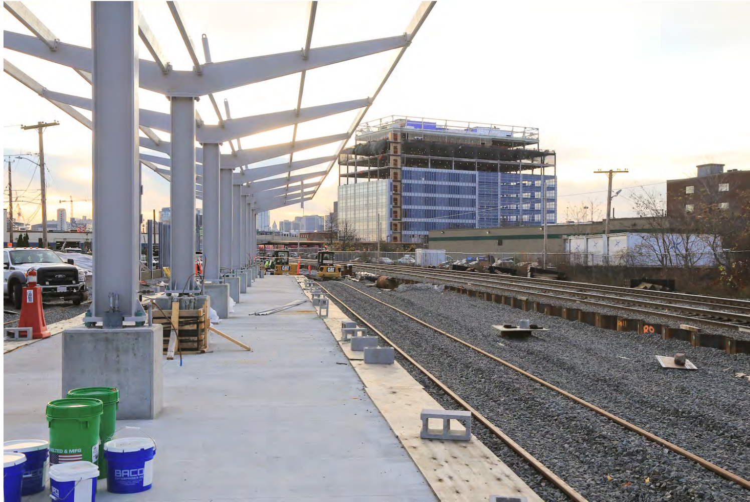
Union Square Station platform. Steel placement for canopy underway. Light rail tracks in place. November - 2020
