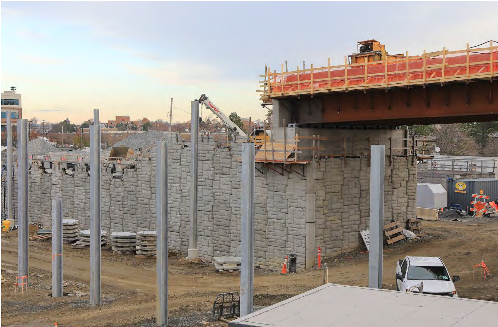
Mechanically Stabilized Earth (MSE) walls near completion - November 2020
