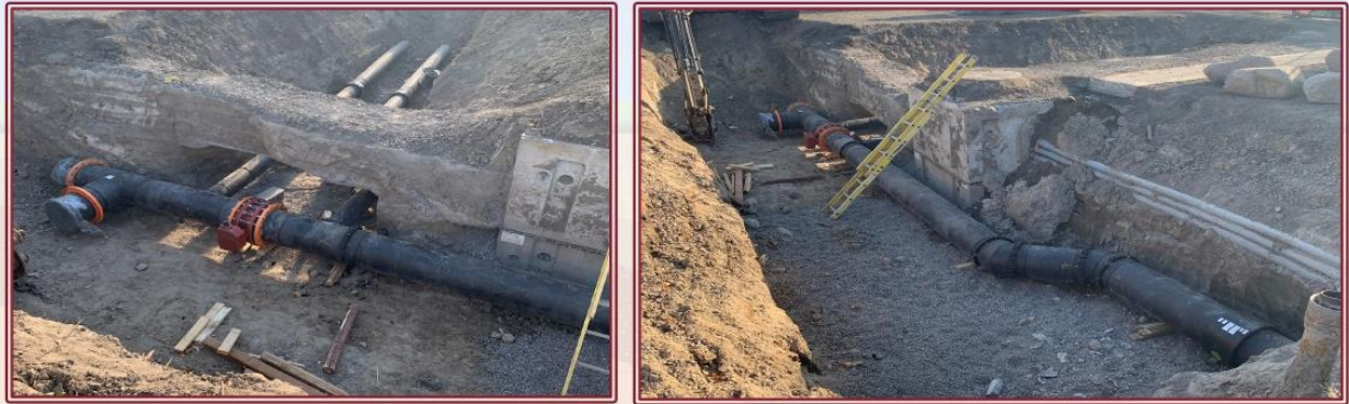
18" diameter HDPE Central Loop
