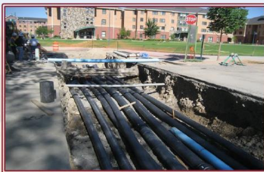
8" dia. Pipes between Central Loop And H.H
