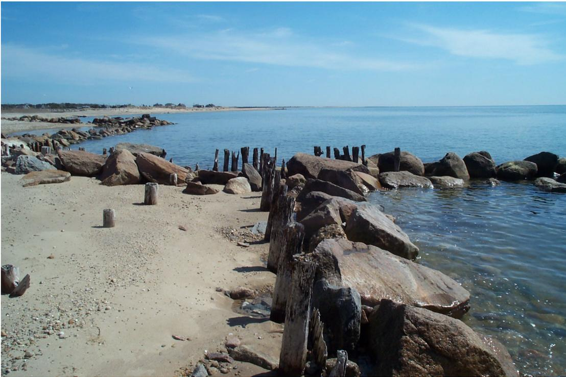
Figure V-5. Photograph of the shoreline west of Menauhant Beach taken in 2004 showing remnants of a timber bulkhead and groin, as well as more recent stone structures.
