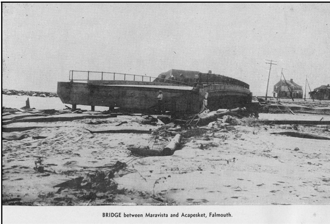
Figure V-6. Photograph of the old Great Pond bridge immediately after the 1944 Hurricane. The photograph shows that storm overwash eroded the roadway and approach ramps to the bridge. Note the Great Pond jetty at the left side of the photograph.
