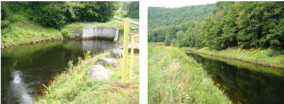
Illustrations 1 & 2: Views of the Canals and Associated Structures
