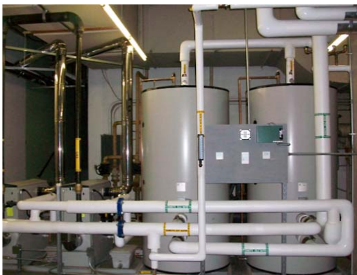
High efficiency gas-fired hot water heaters installed in Medford.
