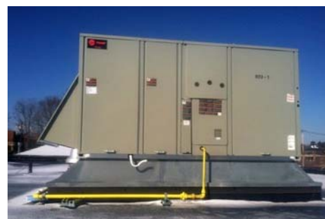
Easton installed higher efficiency rooftop units with energy recovery, part of the HVAC system, at the joint police and fire station.
