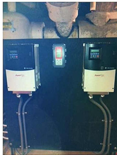
Variable frequency drives (VFDs) installed at Winchester High School.
