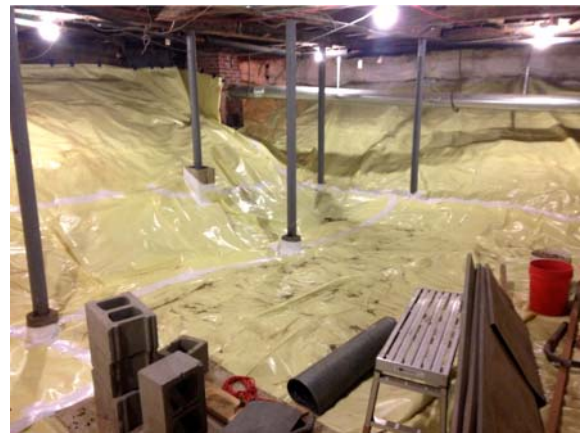
Excavated crawl space under the Ashfield Town Hall with foundation insulated and sealed up.
