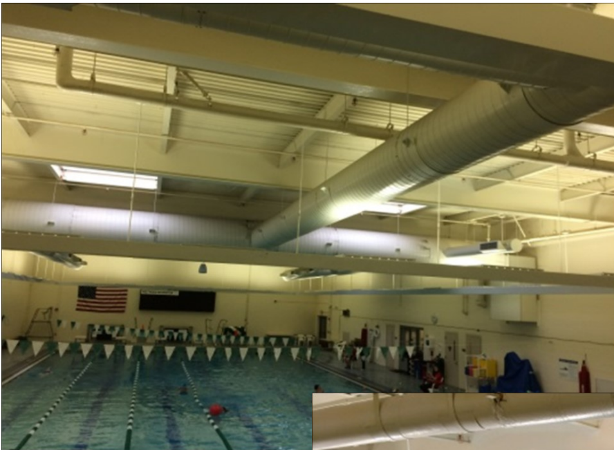
Caption: Before (above) and after (right) the upgrade to LEDs above the pool at the Town of Westwood's High School. The lighting is anticipated to save 33,256 kWh for a cost savings of $5,155 per year. In addition, maintenance costs will be greatly reduced, and visibility will be greatly improved.
