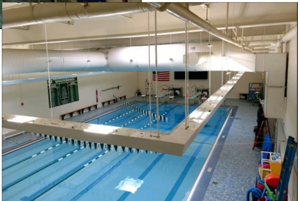
Caption: Before (above) and after (right) the upgrade to LEDs above the pool at the Town of Westwood's High School. The lighting is anticipated to save 33,256 kWh for a cost savings of $5,155 per year. In addition, maintenance costs will be greatly reduced, and visibility will be greatly improved.
