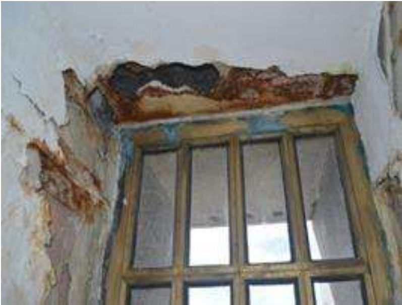
PLASTER FAILS TO STAY ON
