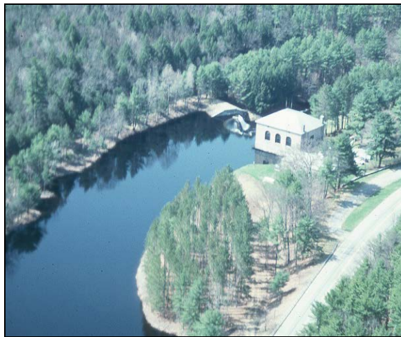
The MWRA's Roger Lonergan Intake on the Ware River
