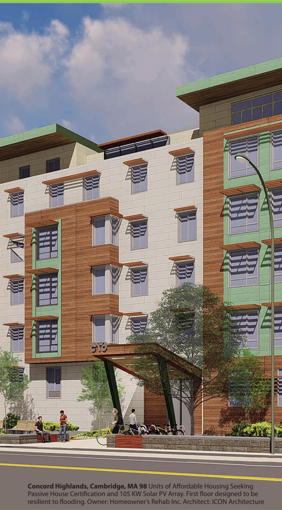
**Concord Highlands, Cambridge, MA** 98 Units of Affordable Housing Seeking Passive House Certification and 105 KW Solar PV Array. First floor designed to be resilient to flooding. Owner: Homeowner's Rehab Inc. Architect: ICON Architecture
