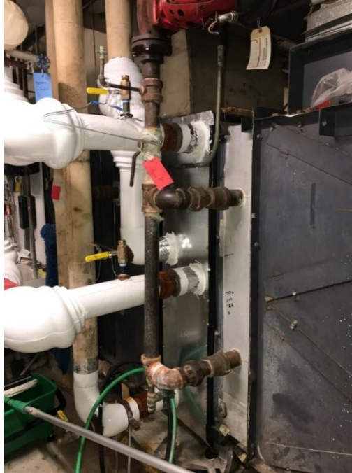
Photo 2 – AHU-1 components, right to left, v-bank filter section, HW preheat coil, CHW cooling coil, HW reheat coil.
