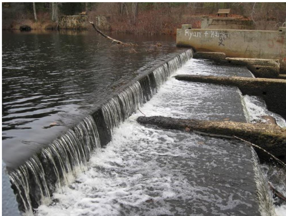
Figure 12: Curtiss Crossing Dam, primary spillway weir (right)
