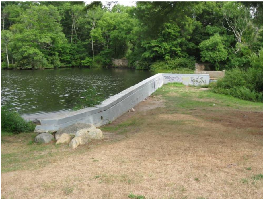
Figure 12: Curtiss Crossing Dam, primary spillway weir (right)
