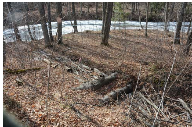
Figure 13. Using logs and brush, a “soft” engineering solution, to control erosion in a maple woods in VT. (Photo Cornell Small Farms Program)
