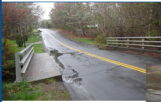
Deficient sidewalks, railing, standing water at bridge joint
