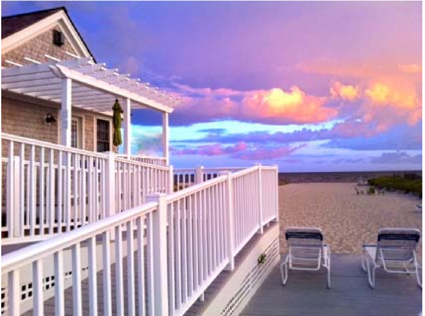
Inn On The Beach – Harwich Port
