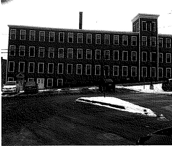
142 Water Street After
