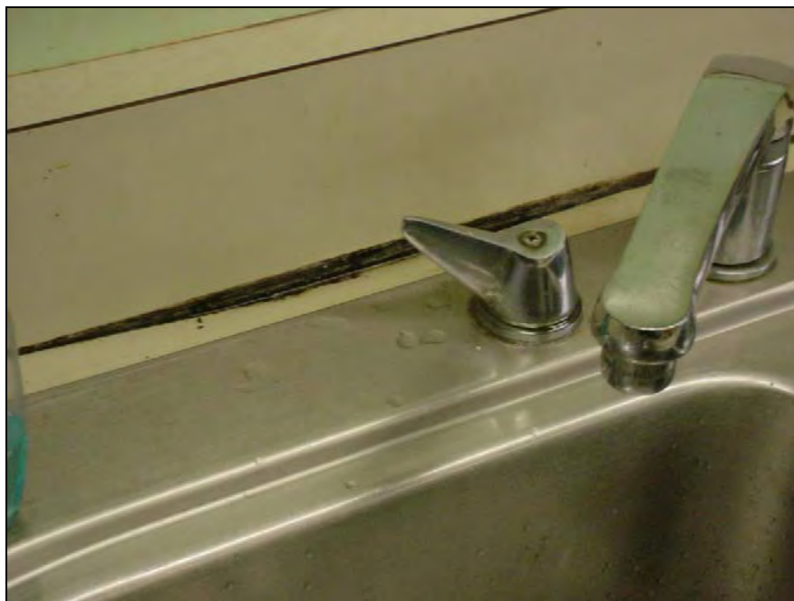
Breach between sink countertop and backsplash with mold growth
