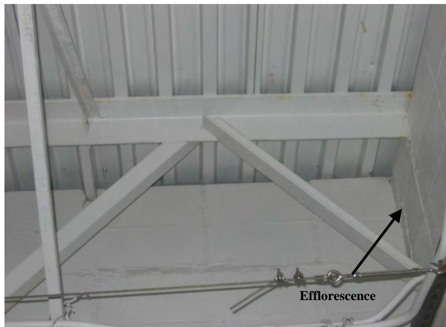
Efflorescence on wall and rust stains on beam, indicating moisture
