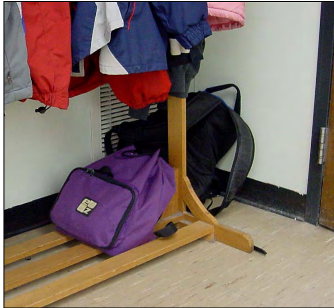
Classroom exhaust vent blocked by items
