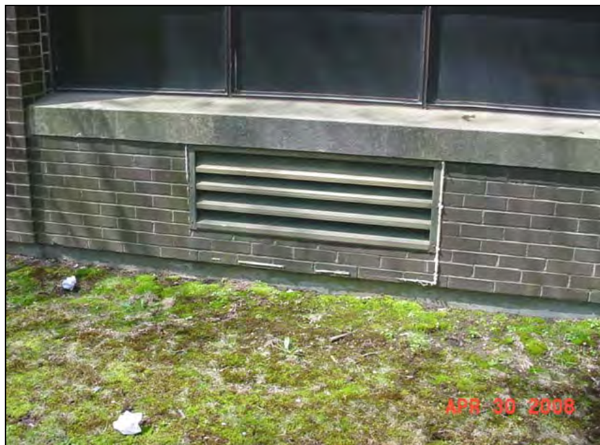
Typical univent fresh air intake
