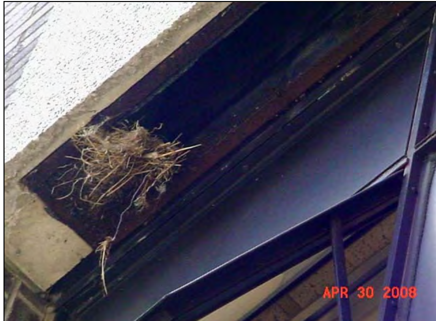
Bird nesting materials in damaged metal grate
