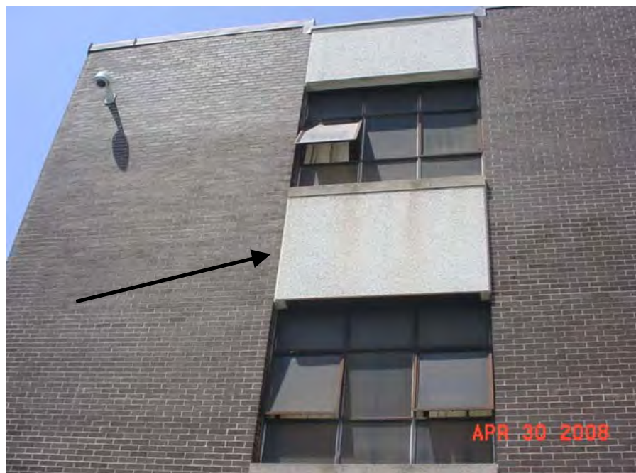
Spandrel wall panel
