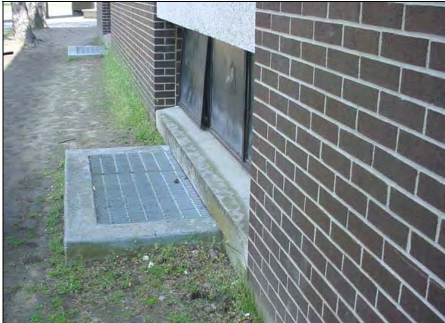
Fresh air intake for some ground floor classrooms
