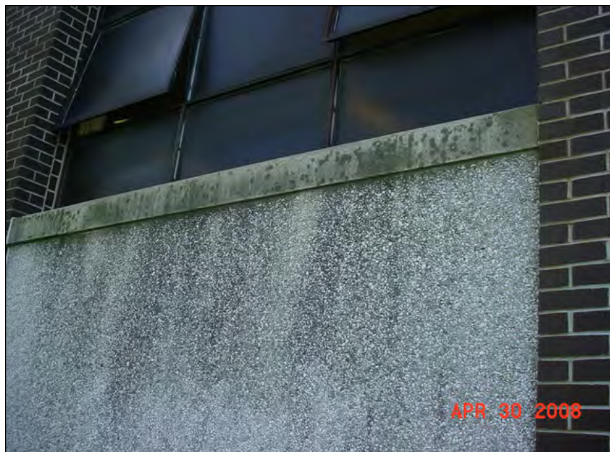
Moss growth resulting from incomplete drying
