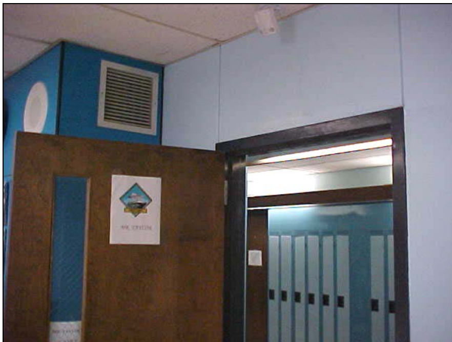
Proximity of classroom exhaust vent to open hallway door
