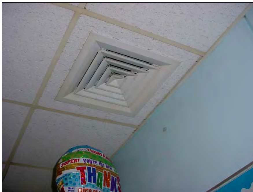
Fresh air supply diffuser
