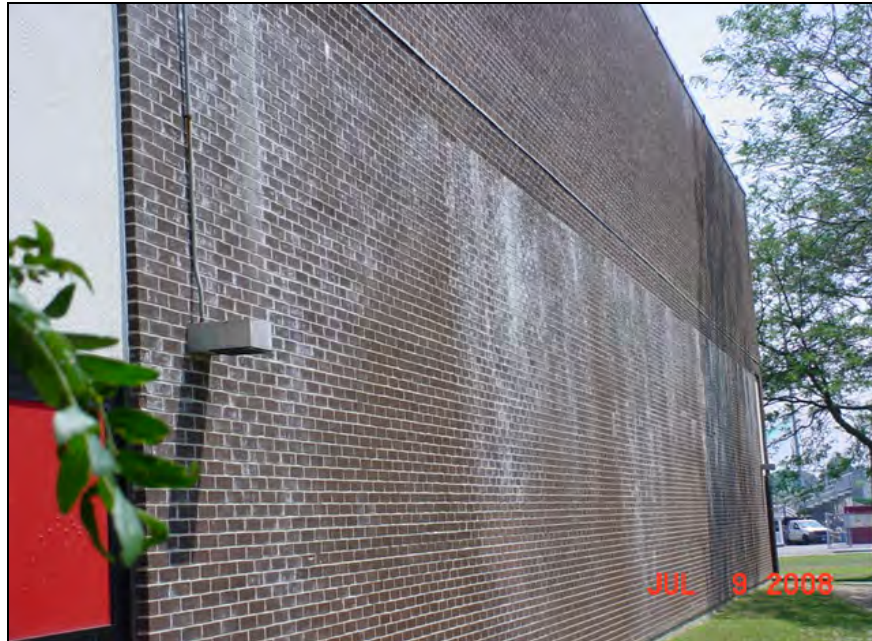
Exterior wall to pool area, note efflorescence line
