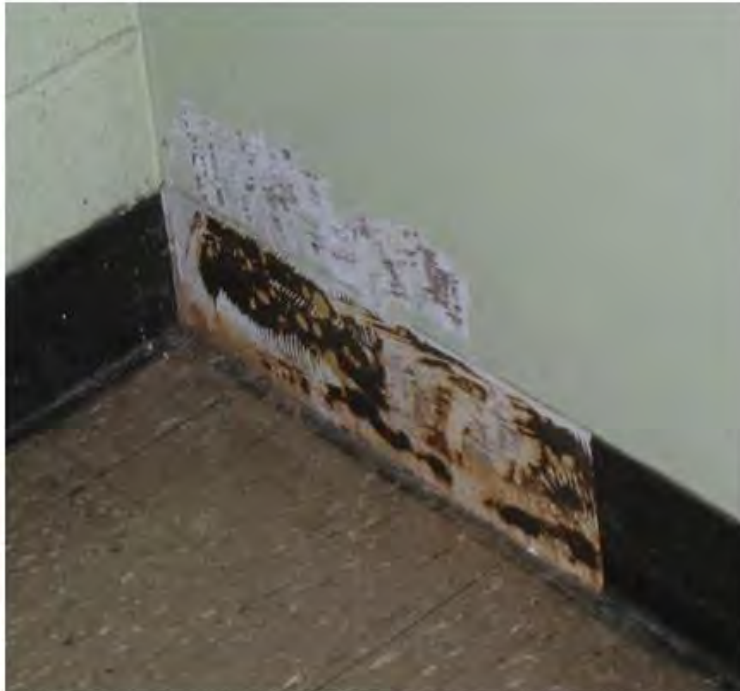
Figure 7c: Photos depicting walls and baseboard areas typical of bulk sampling activities (e.g., adhesives, vinyl cove, paint)
