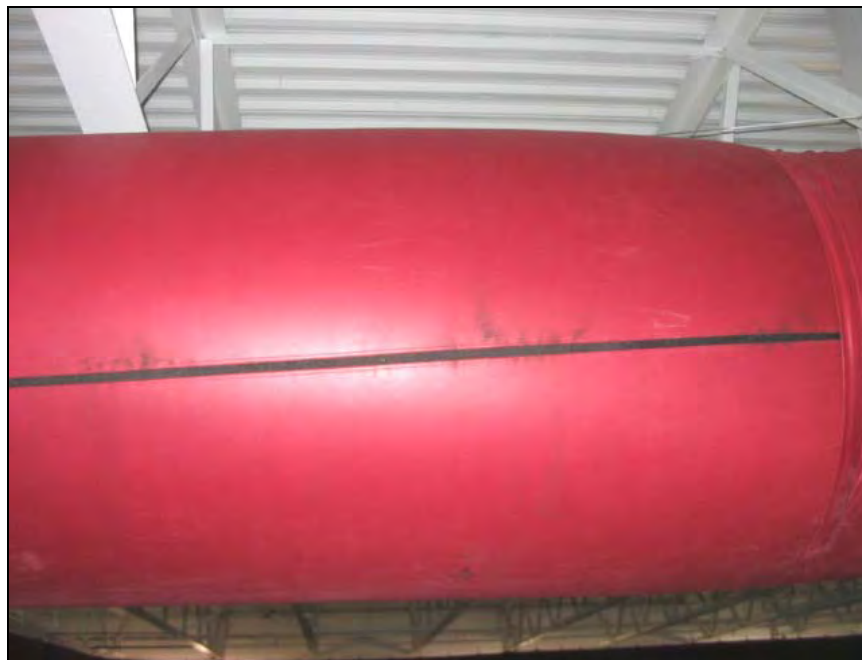
Slotted supply diffuser on supply duct
