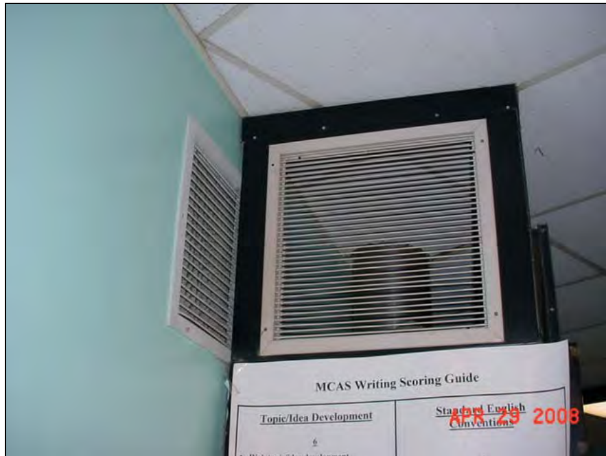
Passive vent on chemical hood adjacent to exhaust vent
