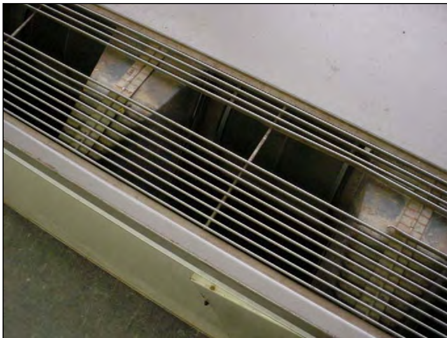
Damaged univent diffuser
