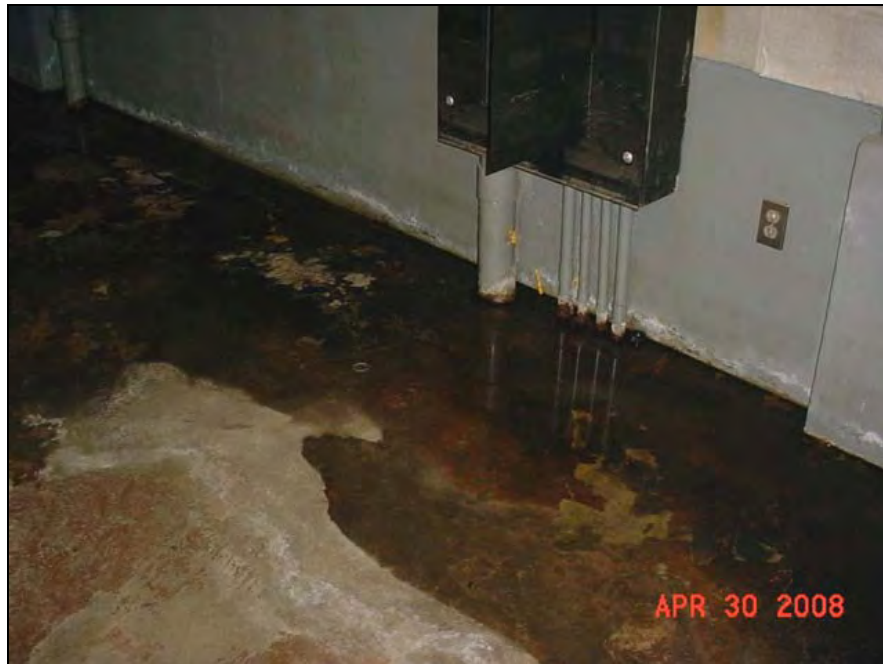
Water around pipes to utility box
