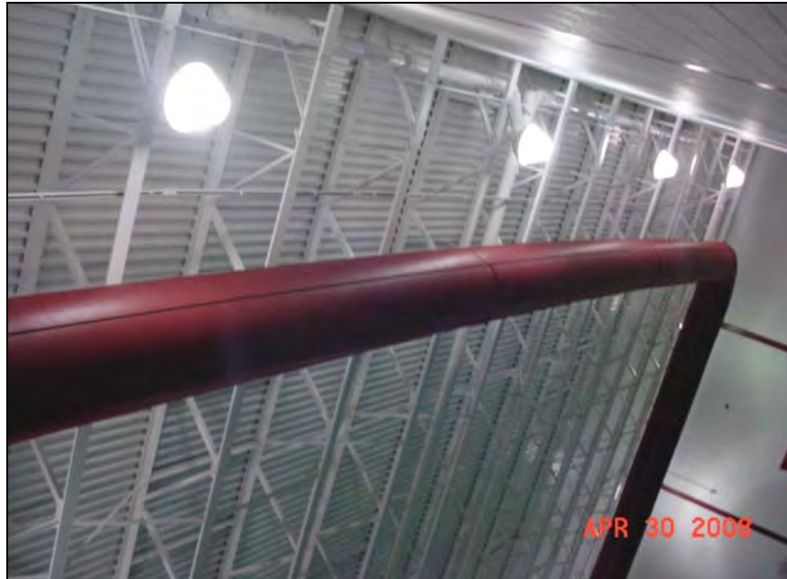
Supply duct for dehumidified air
