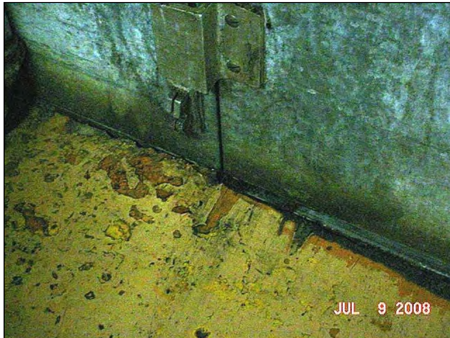
Deteriorating floor near kitchen freezer
