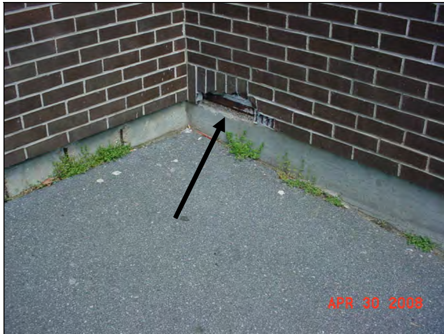
Plant growth around building exterior, also note breach/damaged brickwork
