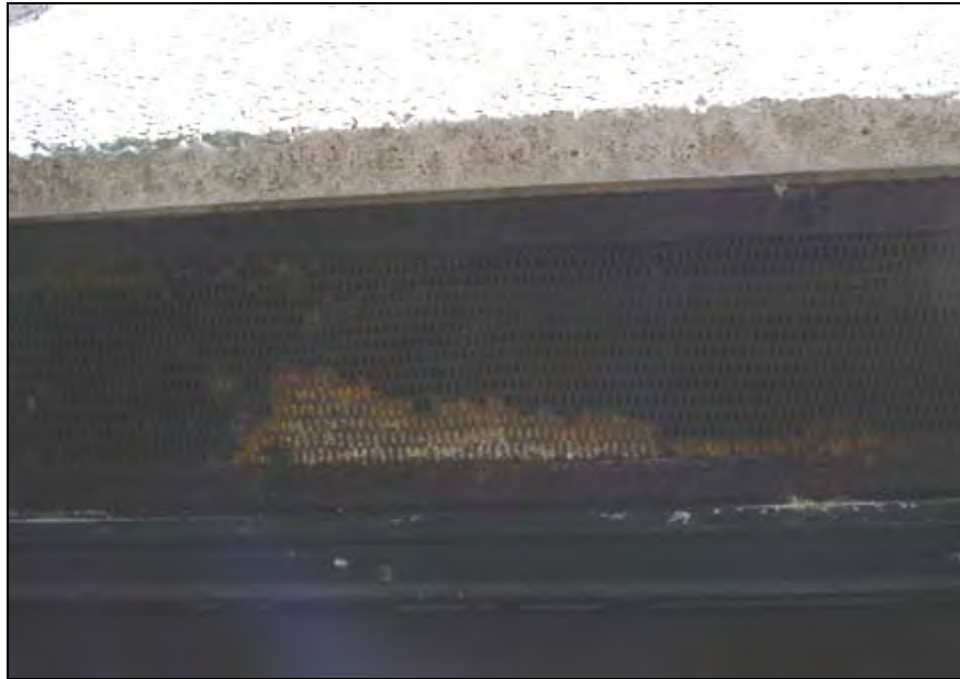
Metal grate between spandrel panel wall and building's exterior wall that allows airflow into univent fresh air intake
