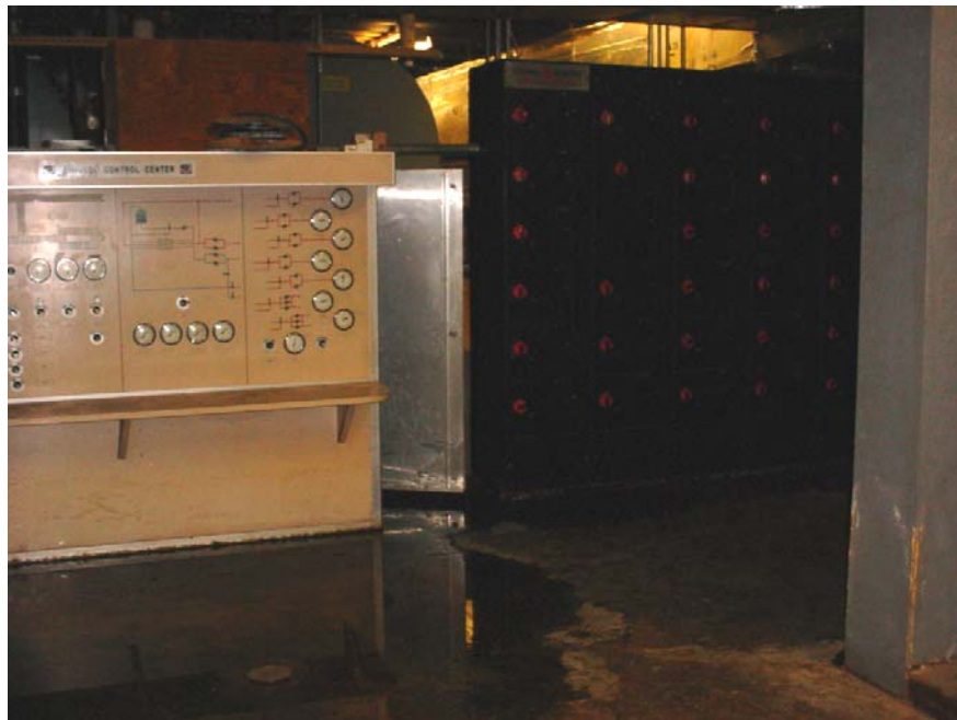
Water in close proximity to electrical panels
