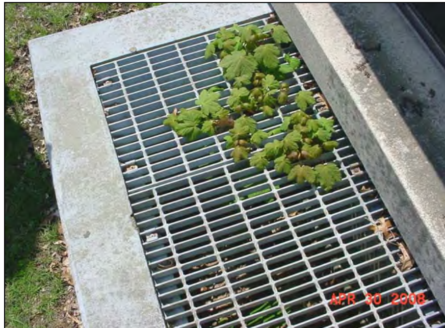
Tree growth in fresh air intake
