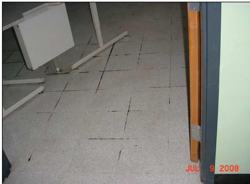
Floor mastic expanding between floor tiles
