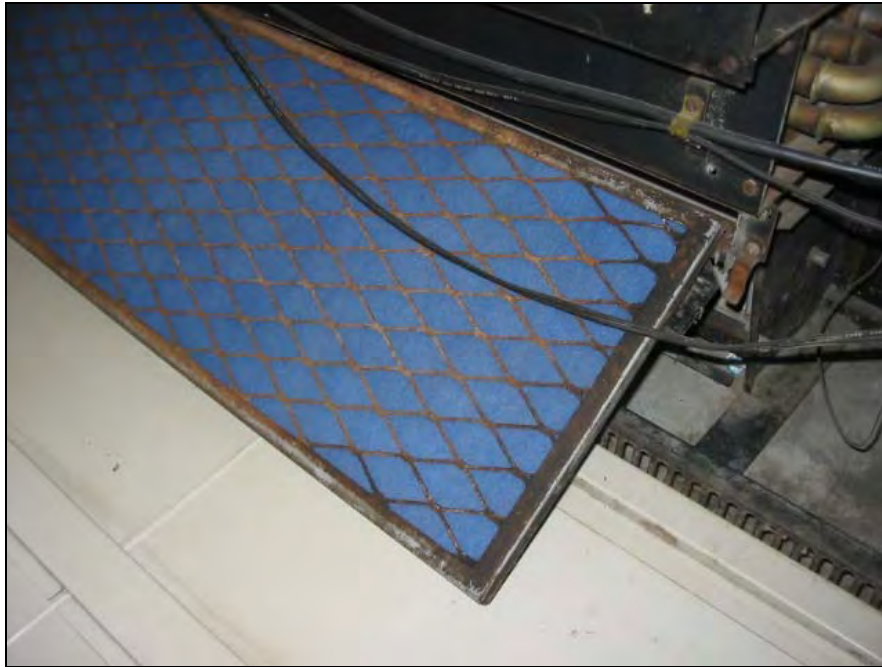
Univent filter (cut to fit media)
