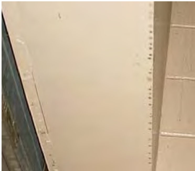
Mold growth on door frame (as indicated by dark spots) between hallway and pool area
