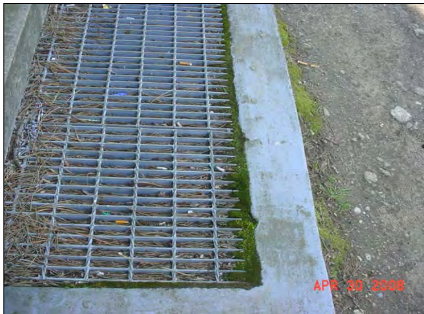
Pine needles, debris and moss growth in/around ground floor classroom fresh air intake
