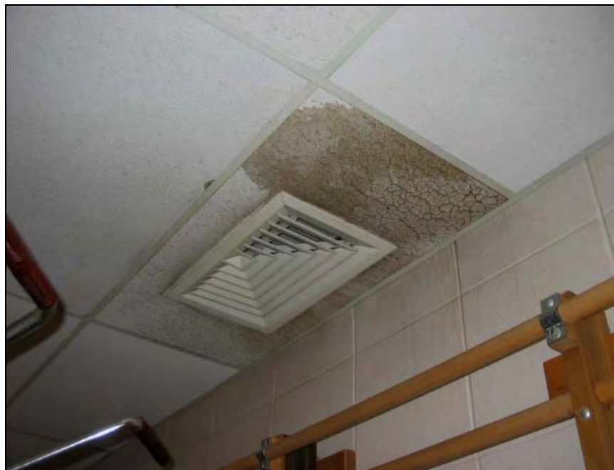
Water-damaged ceiling tile
