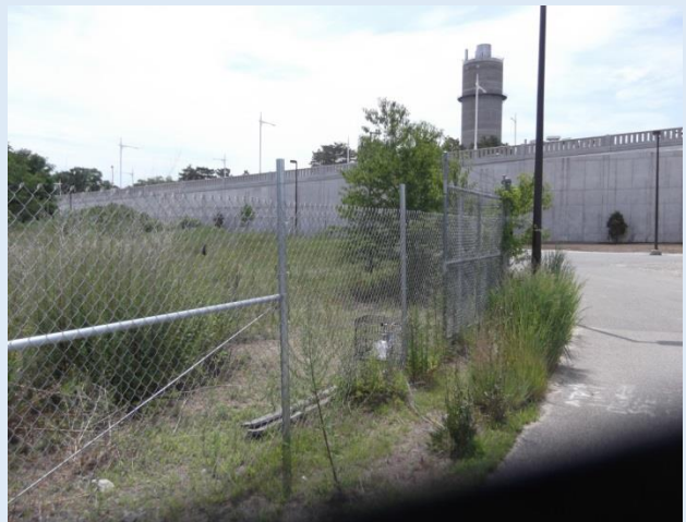
Weymouth 2 – Enbridge Site
