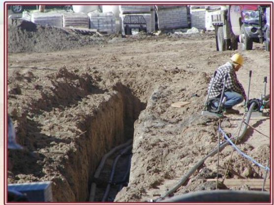
Pipes connecting bore holes
