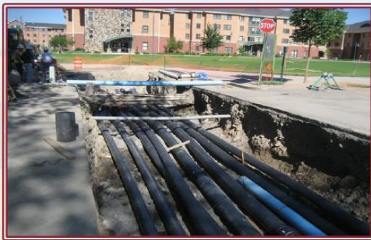
8" dia. Pipes between Central Loop And H.H
