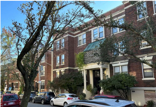
The Allston Brighton Community Development Corporation will retrofit and decarbonize 33 apartments on Carol Avenue in Brighton. (Courtesy of the Allston Brighton Community Development Corporation)
