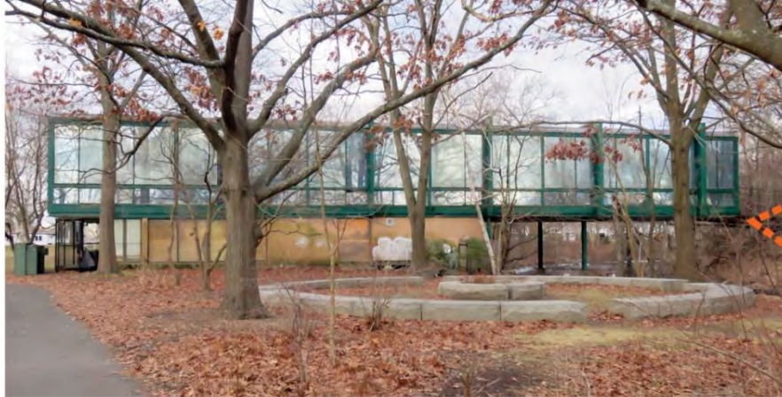
Herter Center with memorial wall
