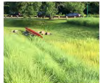
Bioretention area at DCR Community Rowing
