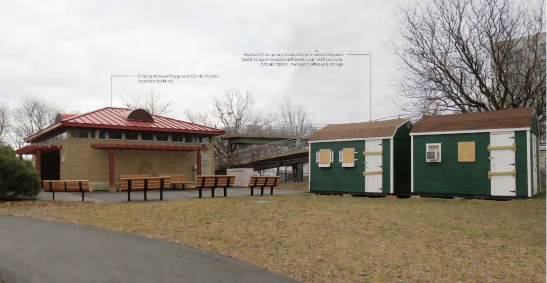
Existing lifeguard break rooms are housed in two temporary sheds.
