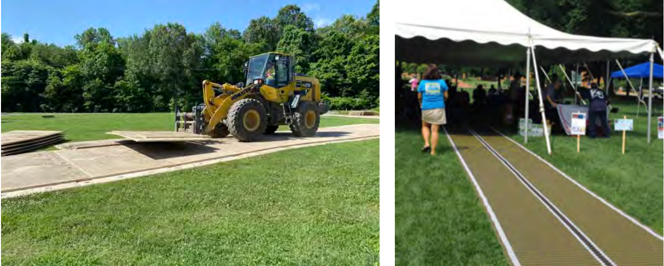
Figure 8. Damage to lawns from intense event usage can be minimized with the use of ground protection mats for vehicles and roll-out accessible mats (Mobi-Mat) for pedestrians.
