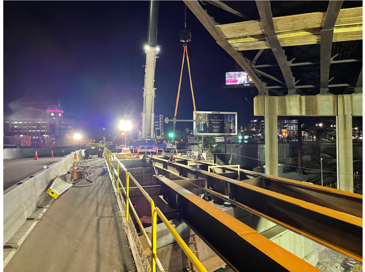
Work during the rail outage, May 9 through May 18, 2025
