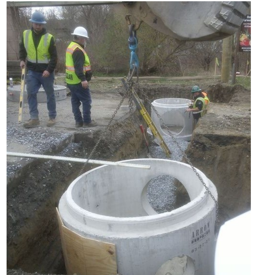
Lanesborough: Route 7 resurfacing Completion: May 2026
