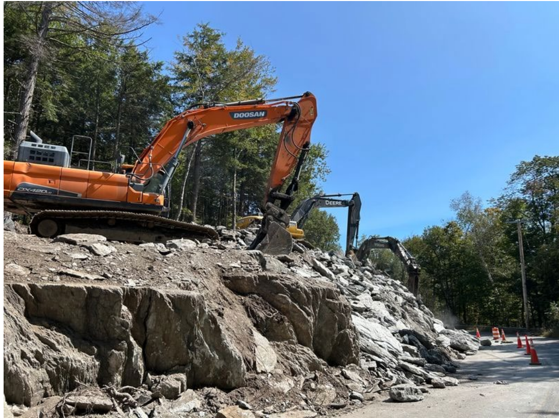
Worthington: construction on Route 143 Bid amount: $16.9 million
