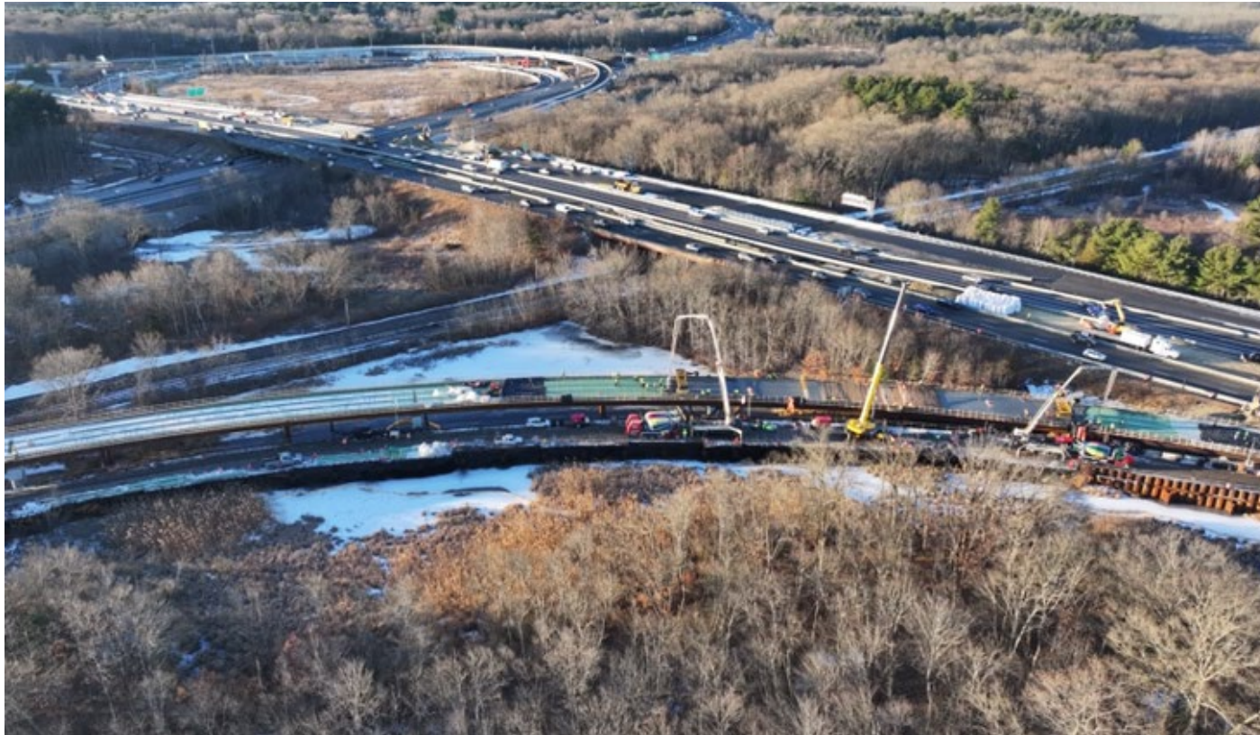
Hopkinton/Westborough: I-90/I-495 interchange reconstruction Bid amount: ~$394 million
