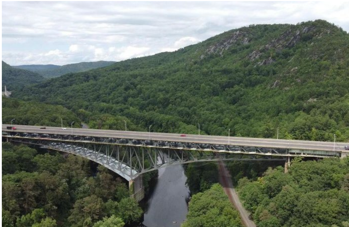
Montgomery/Russell: I-90 over US 20, Westfield River, CSX Completion: May 2026
