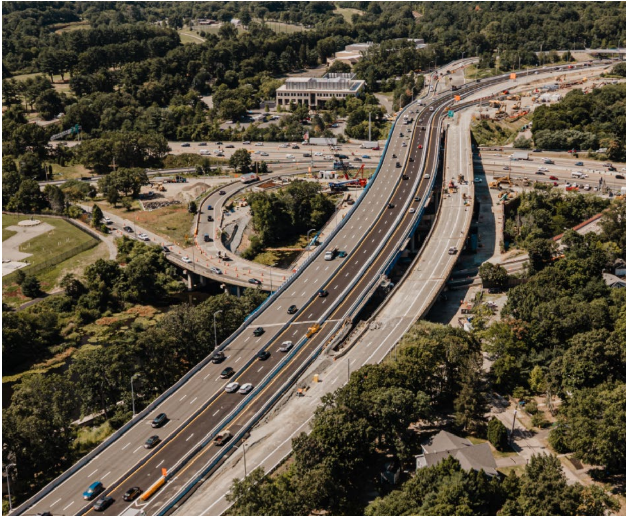
View facing west: traffic on the new I-90 westbound bridge
