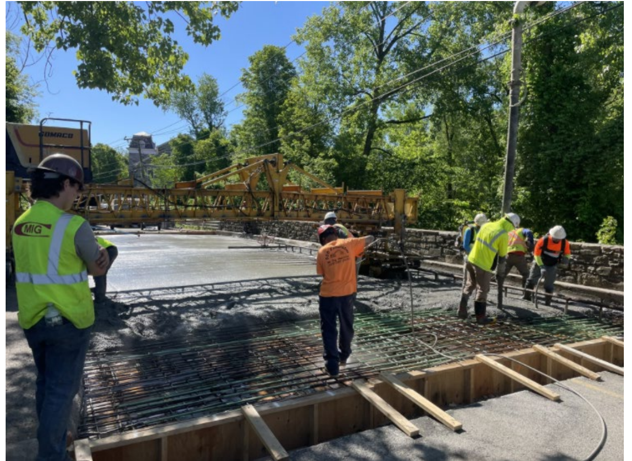
Deck work taking place on East Housatonic Street in Dalton
