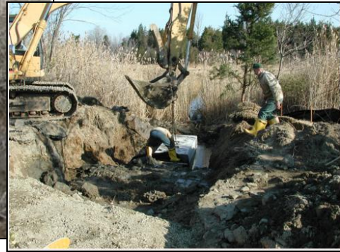
Installation of the new box culvert at Conomo Point. Source: NOAA Restoration Atlas
