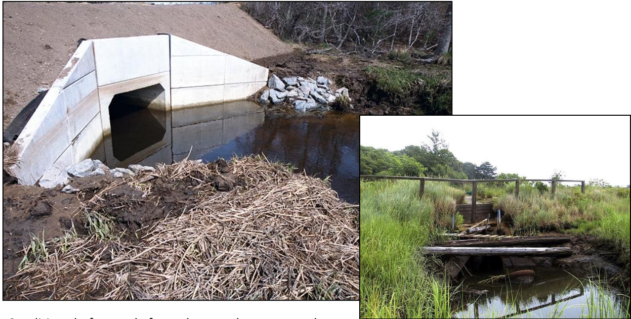
Conditions before and after culvert replacement at the Eastham Bike Path site. Credit: CZM
