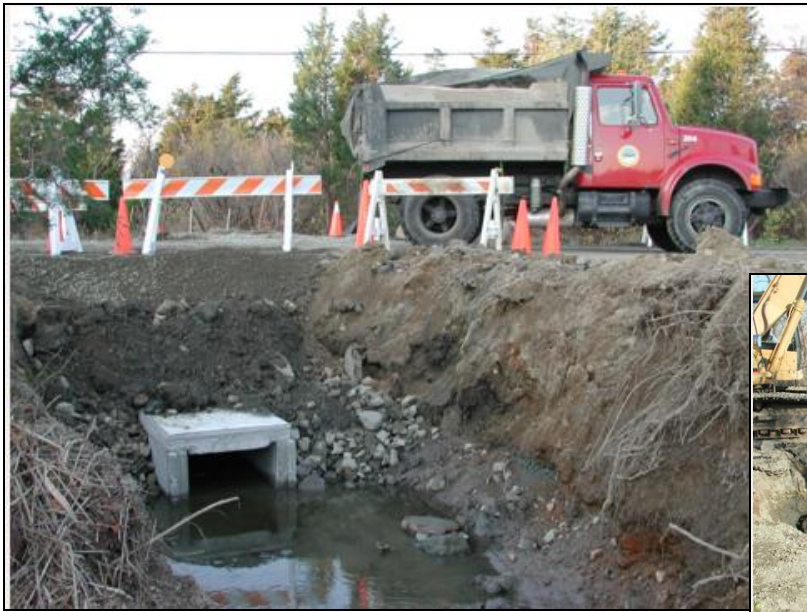
Installation of the new box culvert at Conomo Point. Source: NOAA Restoration Atlas
