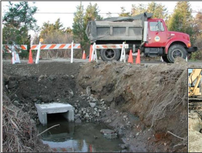
Installation of the new box culvert at Conomo Point.
