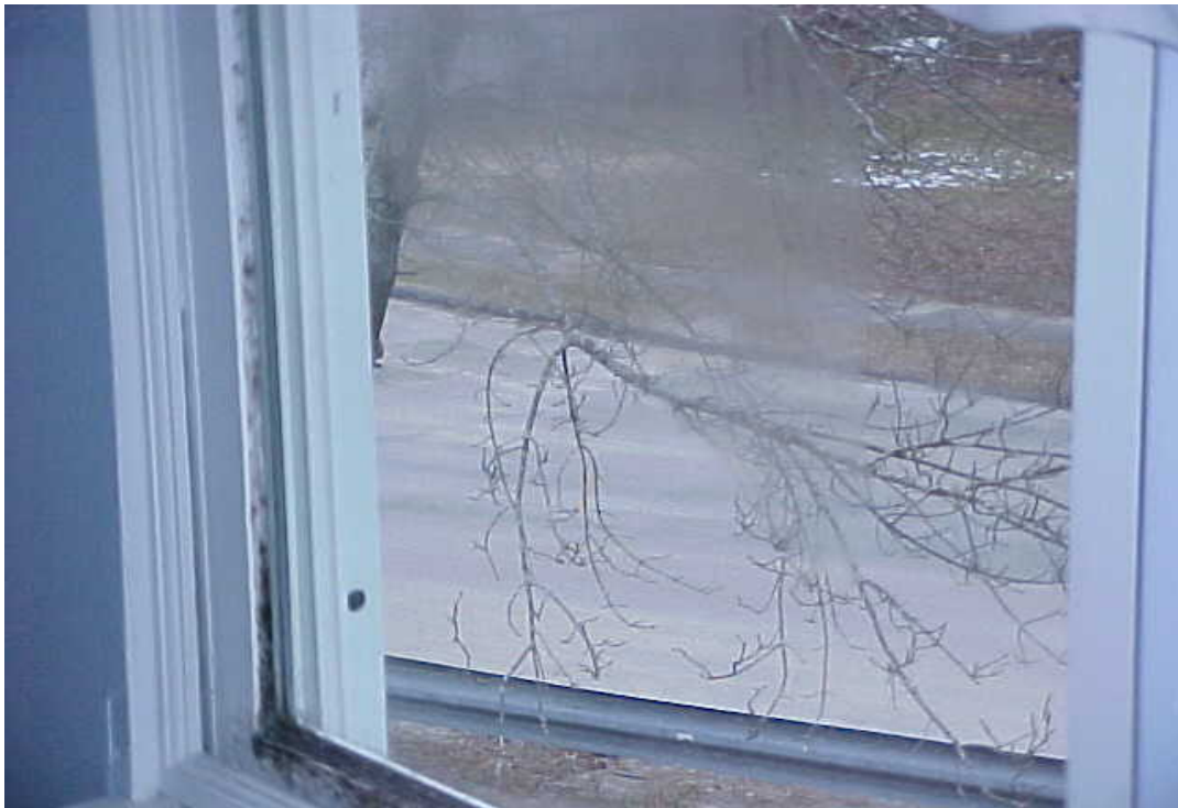
705-1 Family Housing Development, 27 Holbrook Court Bathroom – Window Seal is Broken and Condensation Appears between Window Panes
