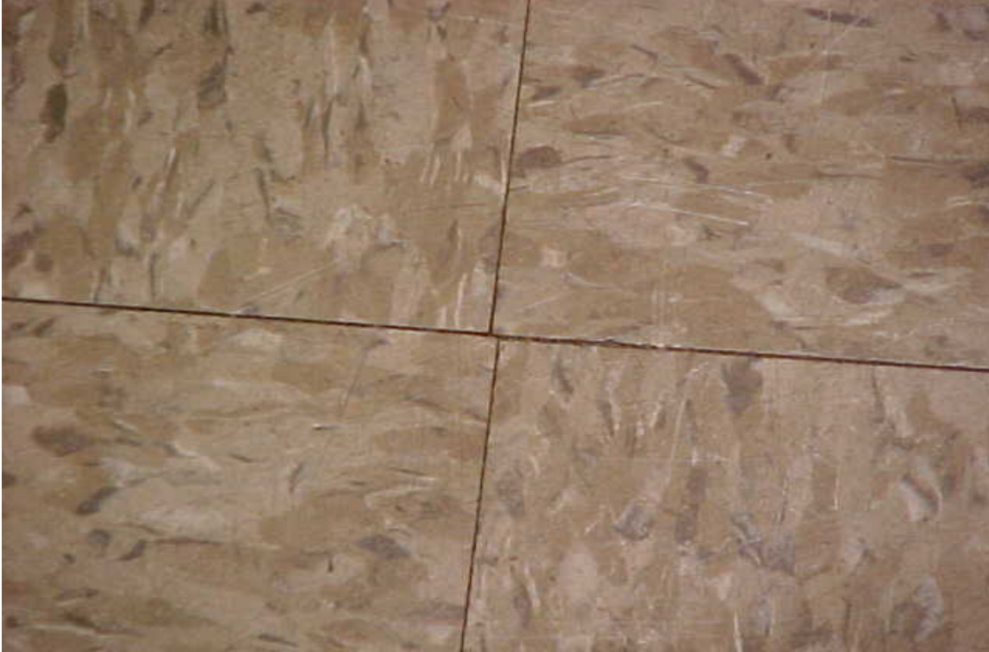
705-1 Family Housing Development, 25 Holbrook Court Living Room – Rehab Contractor Left Residue on Sub-Floor, Sub Floor Settling, Tiles Cracking and Breaking
