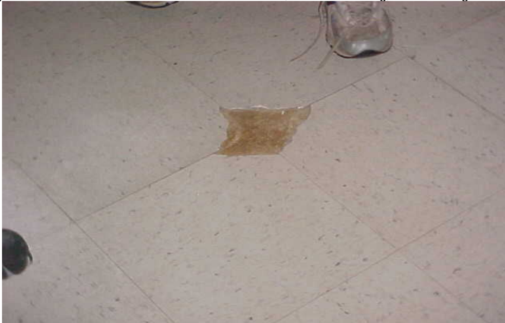
705-1 Family Housing Development, 25 Holbrook Court Living Room – Rehab Contractor Left Residue on Sub-Floor, Sub Floor Settling, Tiles Cracking and Breaking
