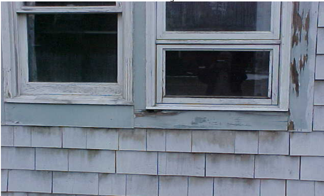
667-2 Elderly Housing Development, 34 Holbrook Court Building Exterior – Rotting Siding and Window Trim, Wood Shingles Splitting and Curling
