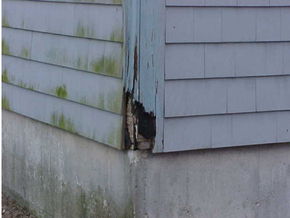
667-2 Elderly Housing Development, 34 Holbrook Court Building Exterior – Rotting Siding and Window Trim, Wood Shingles Splitting and Curling
