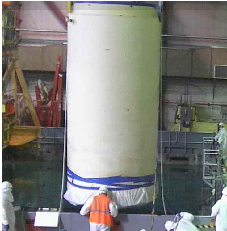
MPC #5 Lowering into Pool
