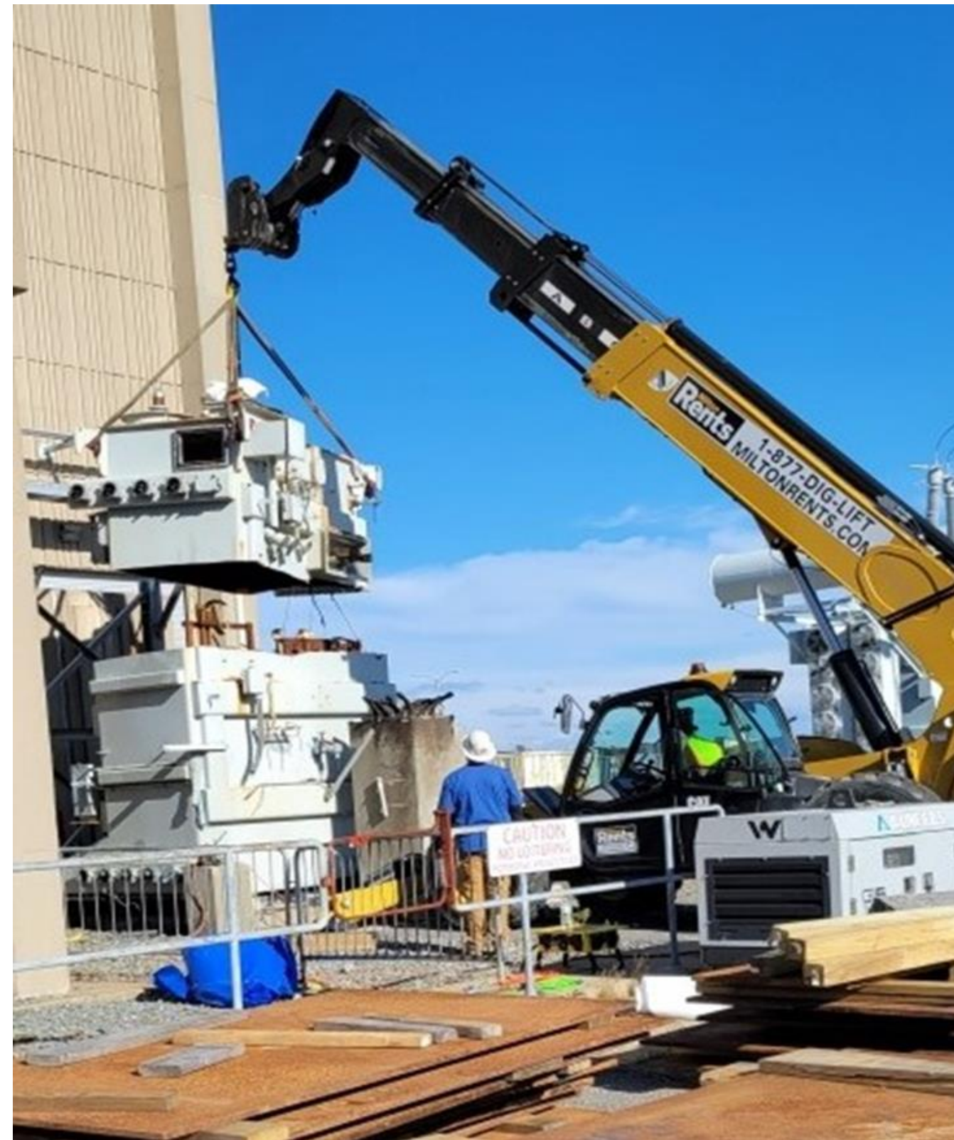
Main Transformer Removal
