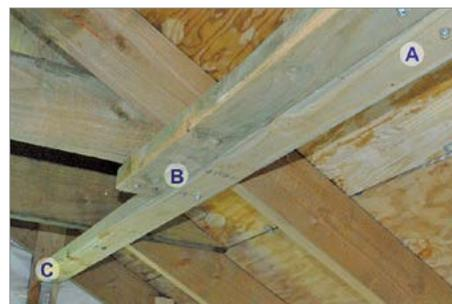
**Figure 4-3.** In this application of lateral bracing, the 2"x4"s are 18 inches from the ridge and connect to horizontal members that attach the opposing trusses. Not all roofs will have the horizontal members. The 2"x4"s are connected with two #14 3-inch screws (A) and overlap over two trusses (A and B). The end is connected to the gable end with an angle or L bracket (C). Image courtesy of Dennis Hwang.
