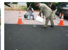
Porous asphalt & permeable pavers
