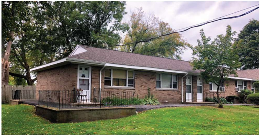
Example: Lee Fort Terrace - Salem Housing Authority is characterized as Small/Medium by wood frame, masonry enclosure, single story.
