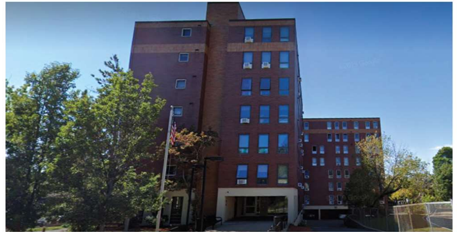
Example: McCarthy Building - Melrose Housing Authority is characterized as Large by masonry frame, masonry enclosure, seven stories.
