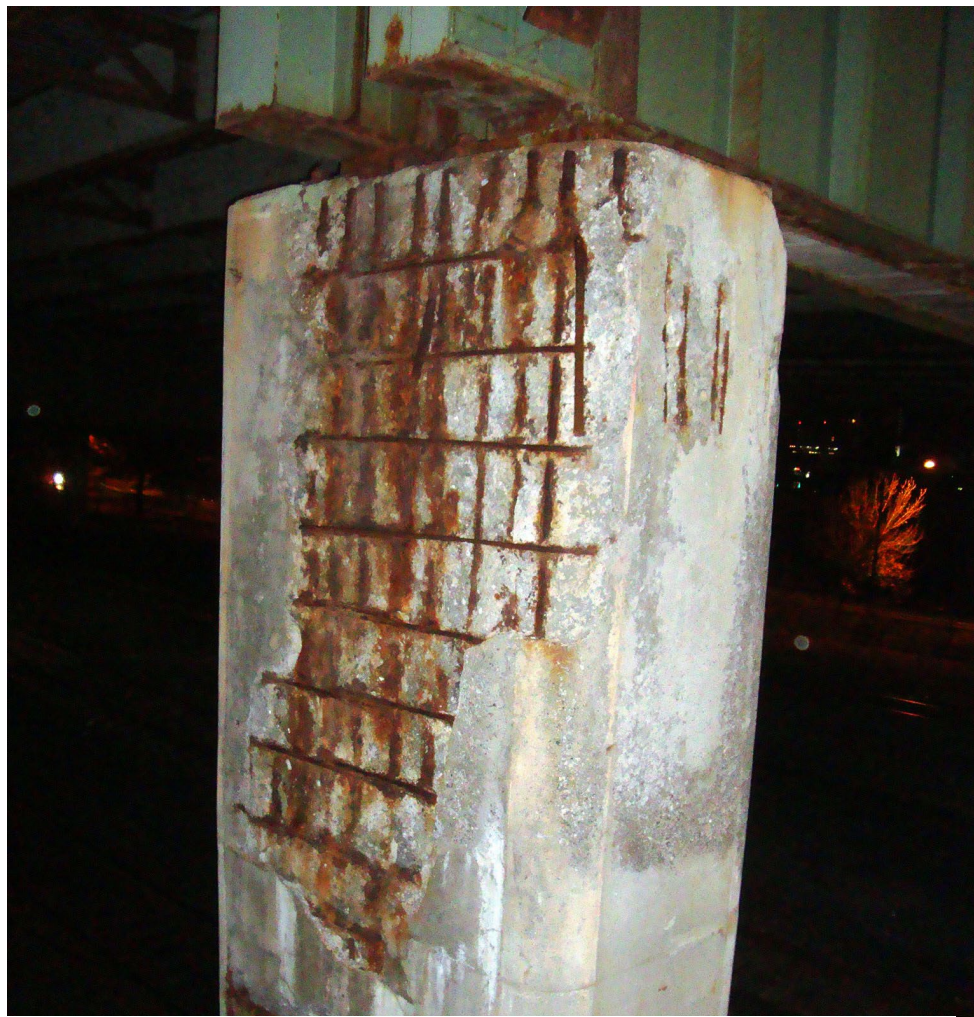
Deteriorated concrete column supporting the I-90 viaduct
