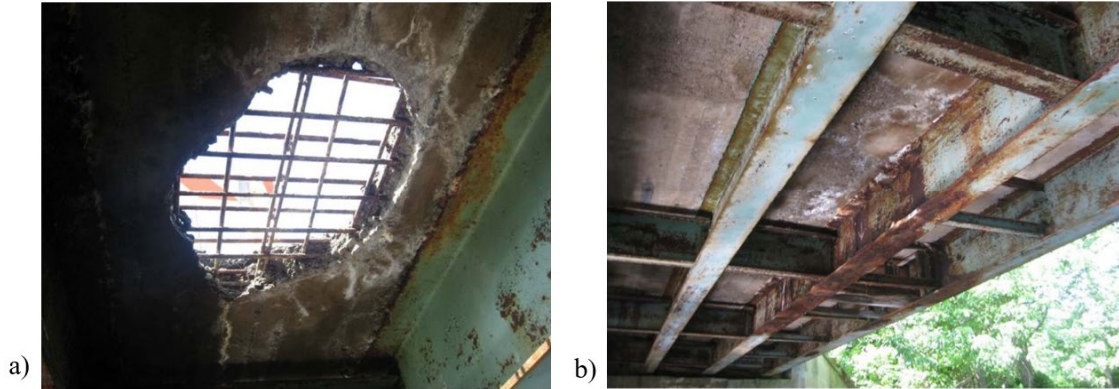
Figure 3.1: a) Hole through the deck and b) map cracking with heavy efflorescence at O-03-009 bridge (adopted from O03009-0TW-MUN-NBI)
