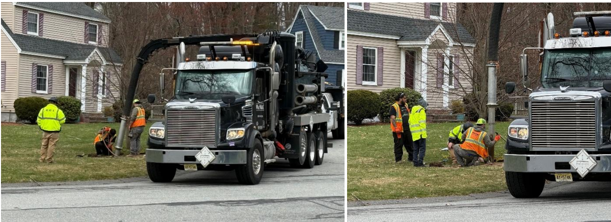
Photo Caption: Town of Andover Conducting Non-Lead Validations. Photo provided by (anonymous) citizen of Town of Andover.
