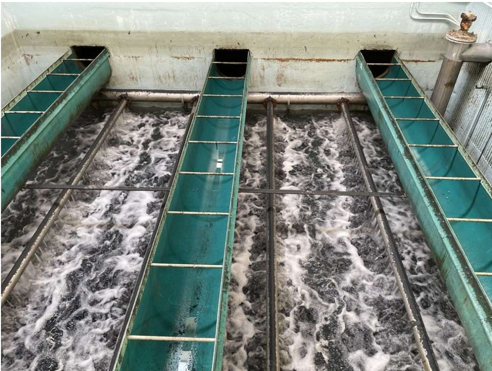
Photo 1: Watching a backwash at the Andover Water Treatment Plant, an 18 MGD surface water treatment plant that serves the towns of Andover and North Reading.
