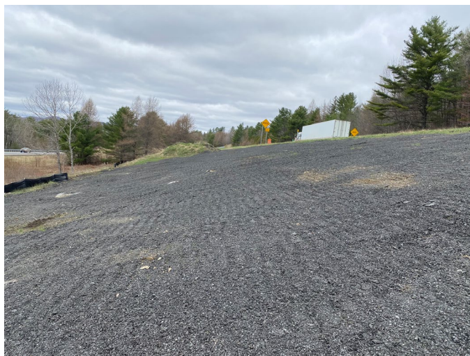
Figure 15: Asphalt millings covering site.
