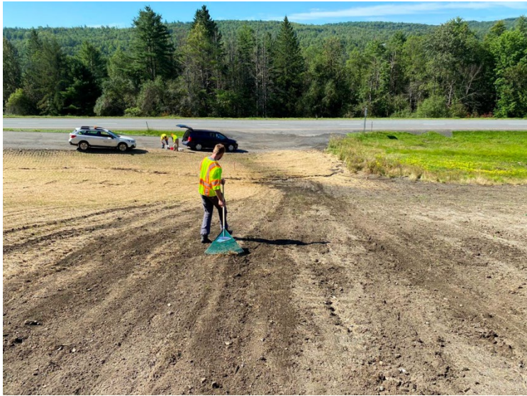
Figure 18: August 22, 2023, Mixing the seed mix and cover crop for broadcasting by hand (left); gently raking seed after broadcasting (right).
