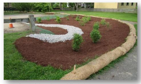
Image 1: Example of a low maintenance infiltration basin
