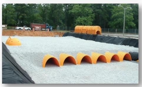
Image 2: Arched chamber subsurface infiltration system, during installation under a parking lot.
