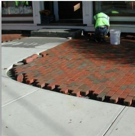
Image 3: Installation of interlocking porous pavers
