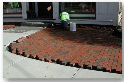
Image 2: Installation of interlocking porous pavers
