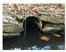
Figure 3. Examples of crossing structures in poor or critical structural condition observed at various locations during field assessments. Left: Degraded headwall; Center: Critical level of blockage; Right: Deteriorated pipe invert.
