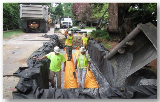
Image 1: Installation of subsurface infiltration chambers under one lane of a municipal right-of-way in Rhode Island.
