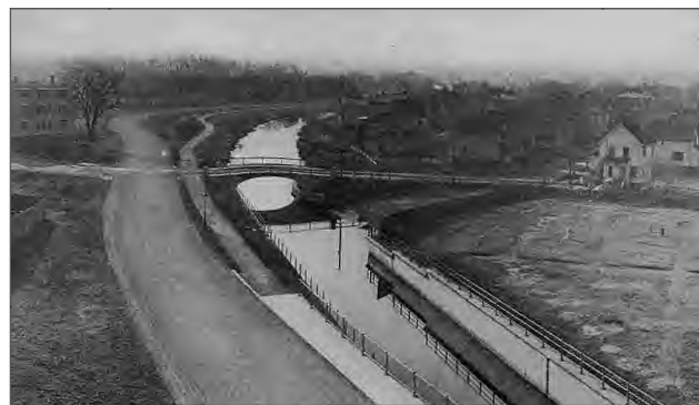
FIGURE 11. The Alewife Brook Parkway and Henderson bridge shortly after construction in 1916
