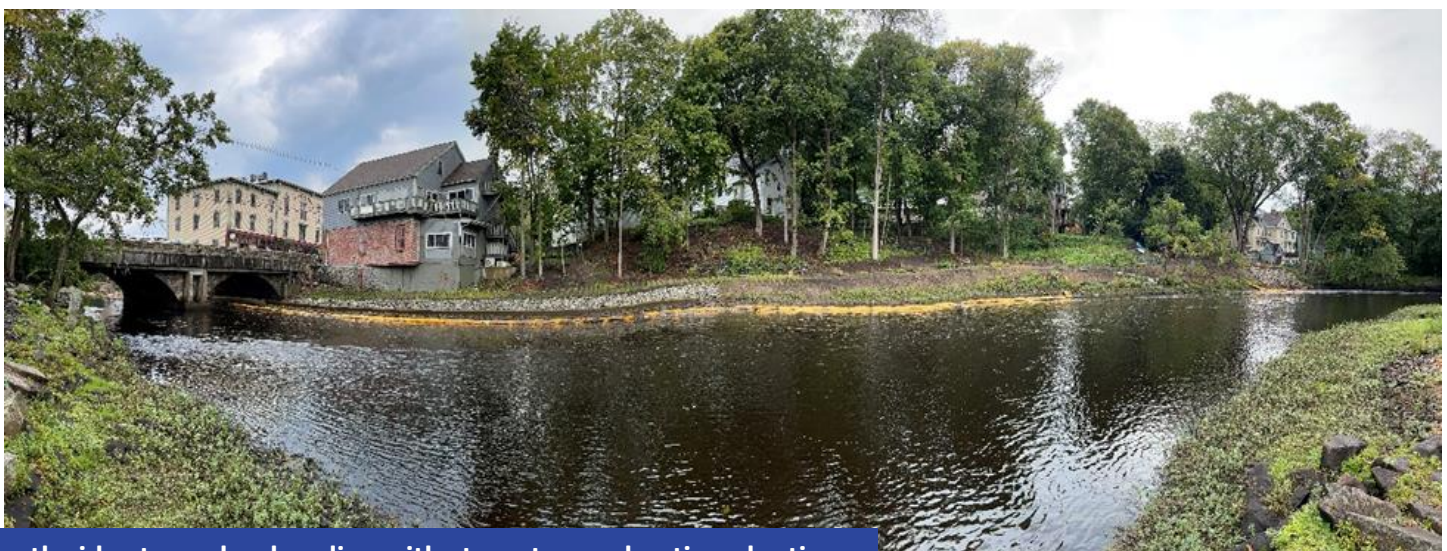
North side streambank radius with stone toe and native plantings
