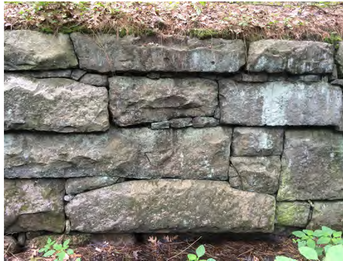
Detail of the 0.25 mile dry laid stone crib wall under and west of Prospect Street.
