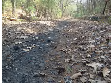
West of Prospect Street: ballast is cupped in the middle of the railbed.
