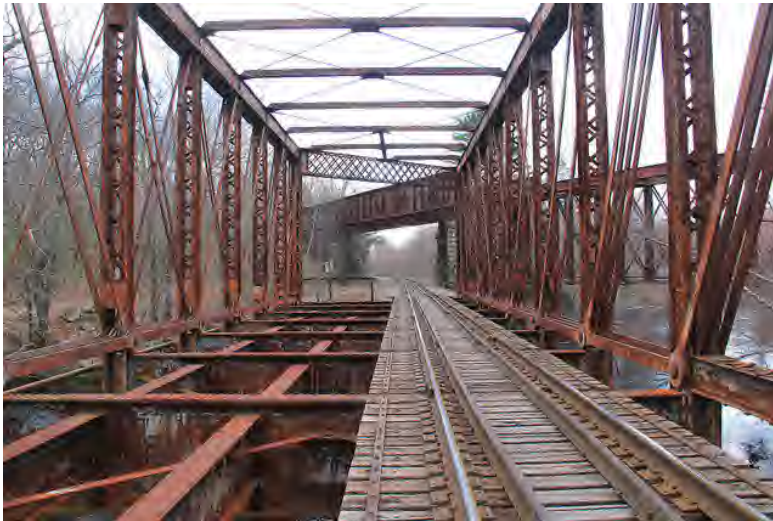
Built in the late 1800's, the Triad crisscrosses the Blackstone River at three different heights to allow three railroad lines to intersect and cross the Blackstone River.
