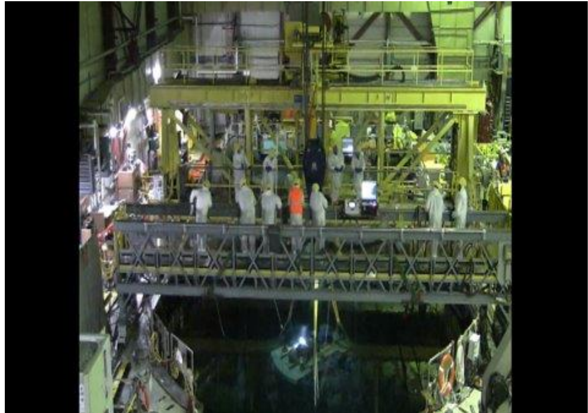
Installation of shroud segmentation tooling
