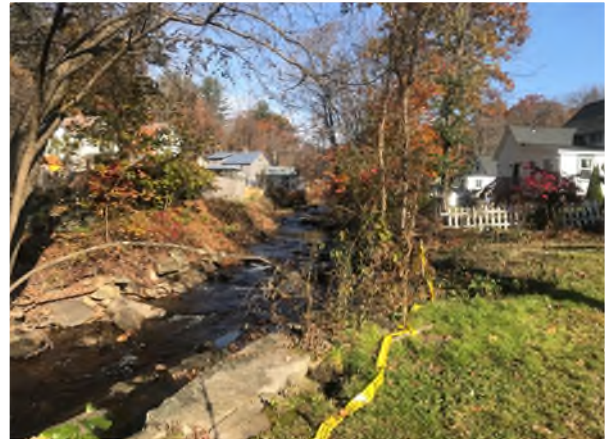
Figure 4d: Bank erosion in lower left corner at Church Street residence, facing north; note the hole in the lawn behind the retaining wall
