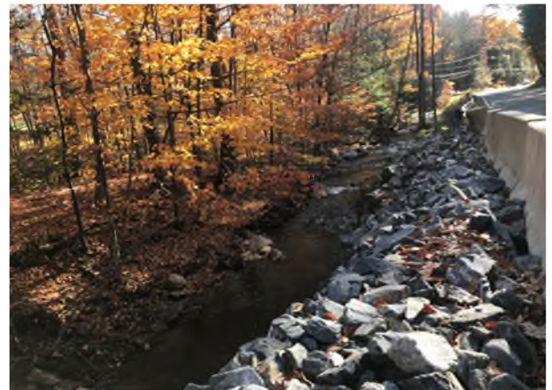
Figure 4f: Riprap placed along North Street after extensive damage to road shoulder, in which bank erosion came within three feet of a sewer main; the former Swamp Road bridge abutments are in the photo background
