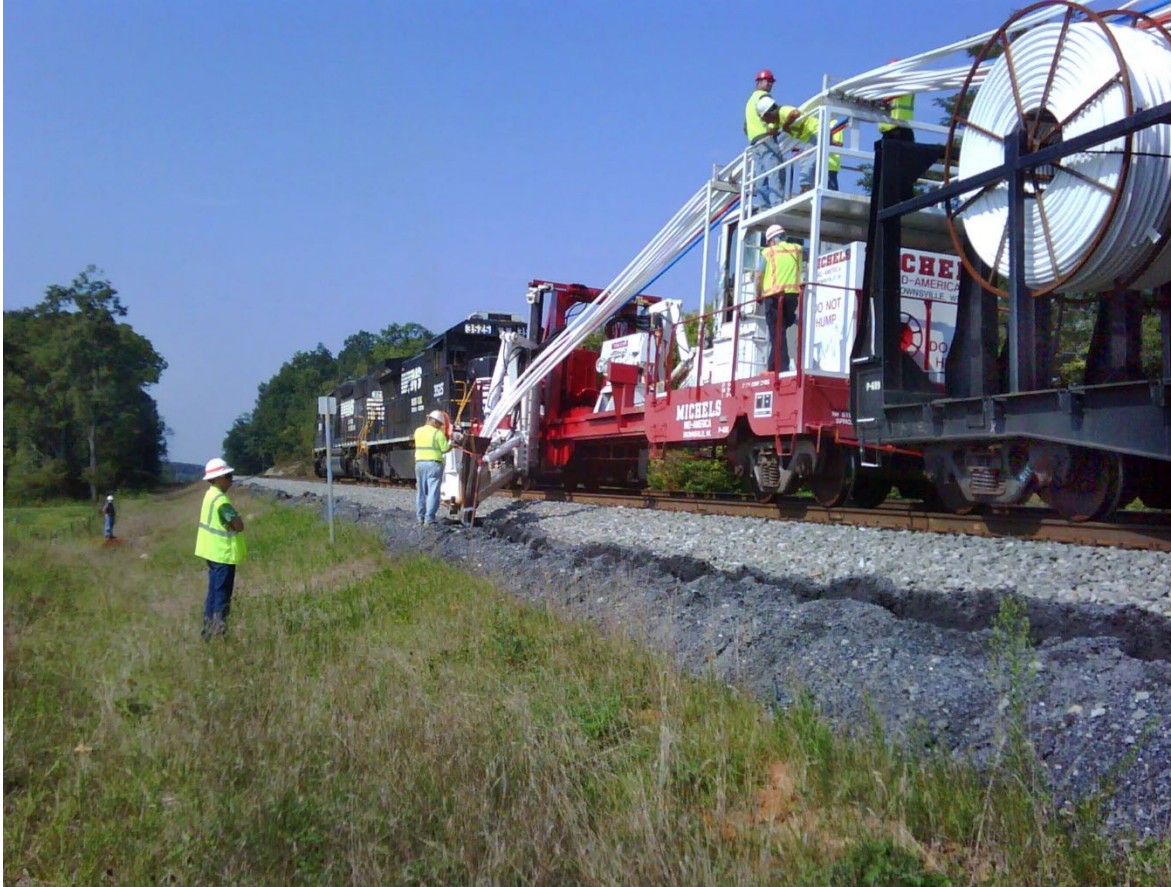
Cable conduit is installed via rail plow in this example photo. Photo credit: Sarasota Herald Tribune, 2010
