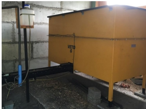
Figure 2 - The hopper and wood chip auger/conveyor
