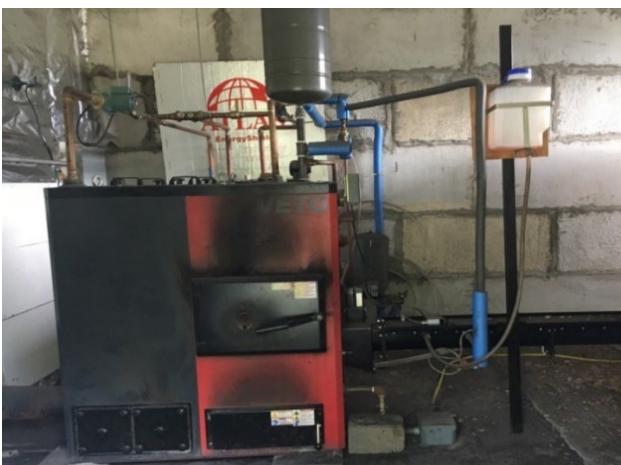
Figure 1 - The boiler/furnace and the auger/conveyor
