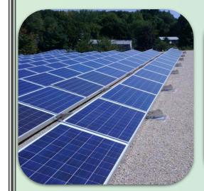
The City has 935kW of behind-the-meter solar PV and is working to more than double this number in the next year. A study completed in 2023 identified 4.6 MW of solar potential across 14 City properties, 1.7 MW of which is on solar-ready roof structures. The City has secured SMART blocks and filed interconnection agreements for these sites.
