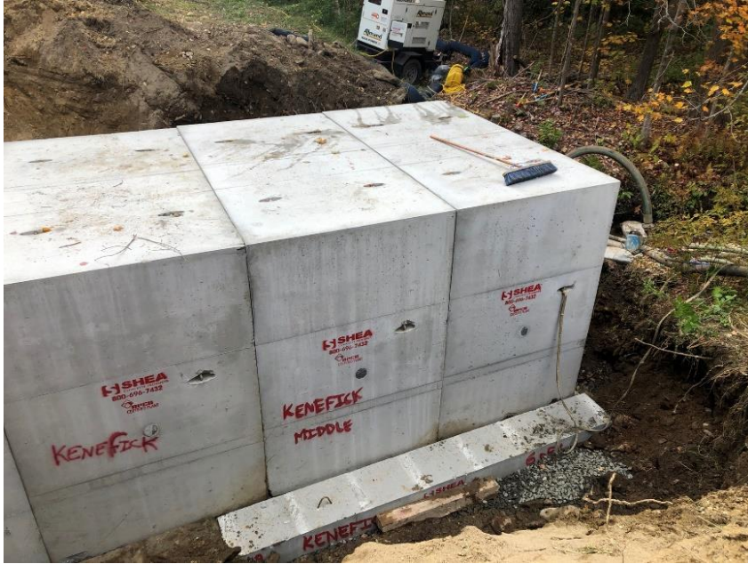
All pieces of the culvert body in place
