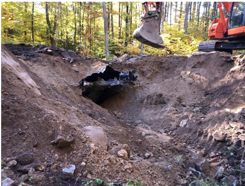
Taking out the old culvert
