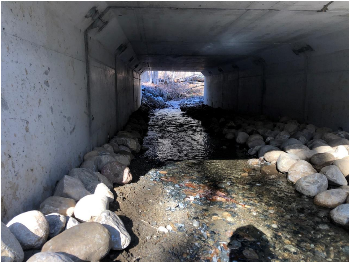
New streambed in new culvert
