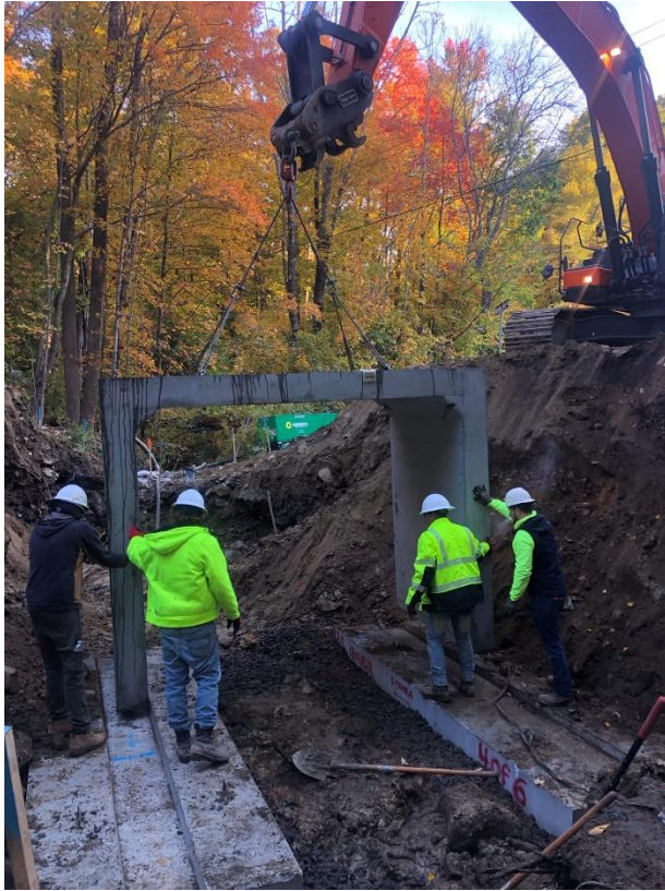
First piece of new culvert on footings
