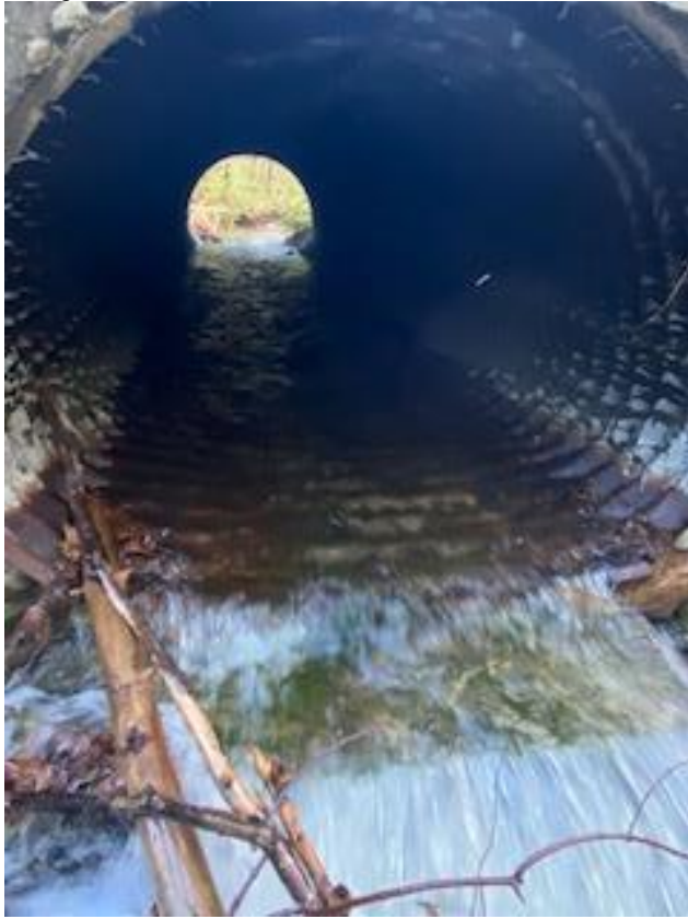
Culvert with pool before replacement
