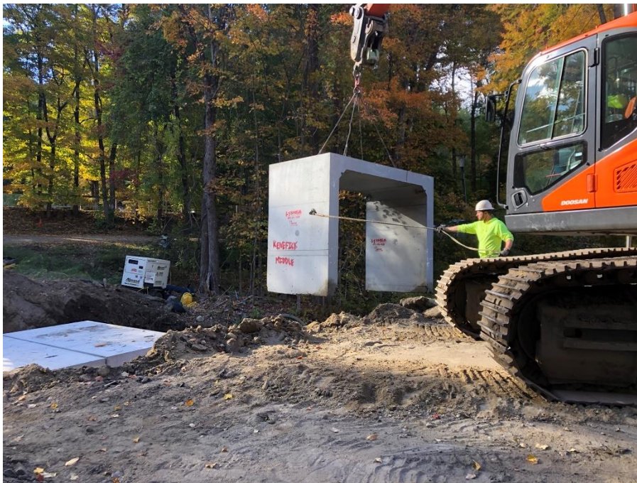
Third piece of new culvert going in
