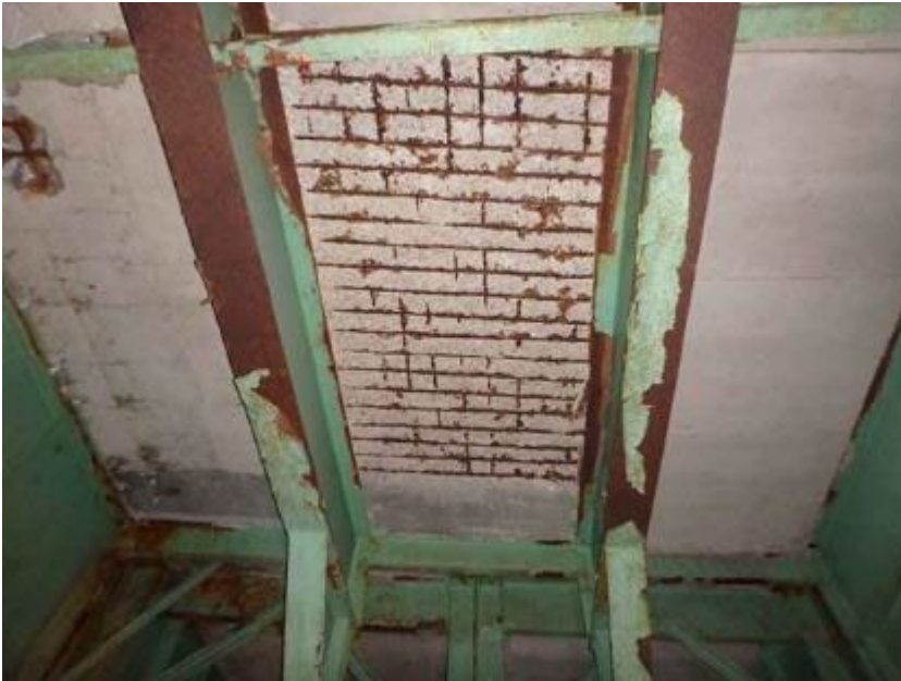
Deteriorated Bridge Deck and Heavy Rust on Girders
