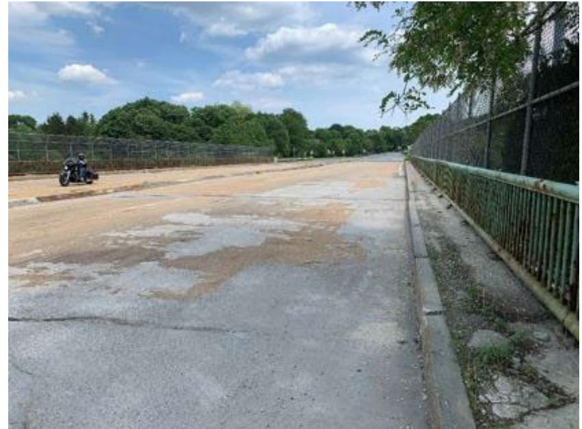
Deteriorated Riding Surface, Rusting Bridge Rail, No Bicycle Accommodations and Settling Sidewalk
