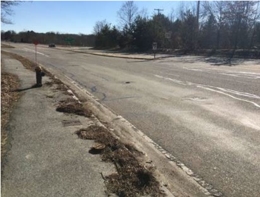
Overgrown Sidewalk, Deteriorating Curb and Pavement
